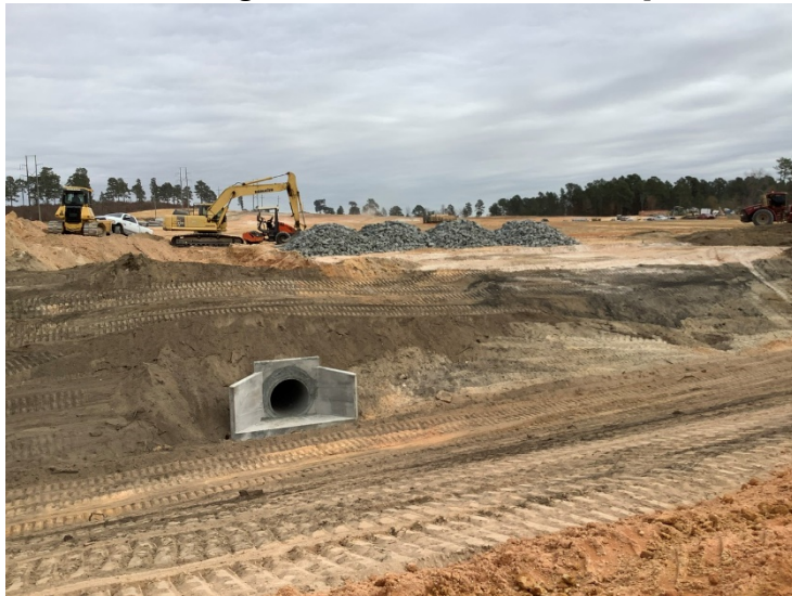
Site – View looking East – Detention Pond 2 [12.07.2021]
