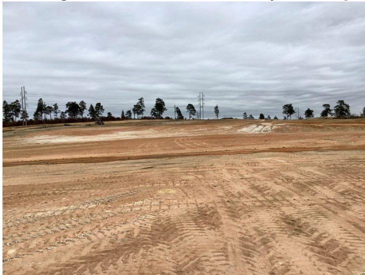
Site – view looking North [12.07.2021]
