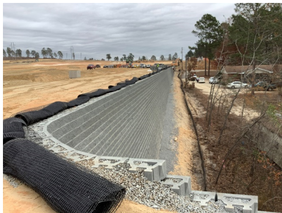
Site – South retaining wall view east [12.07.2021]
