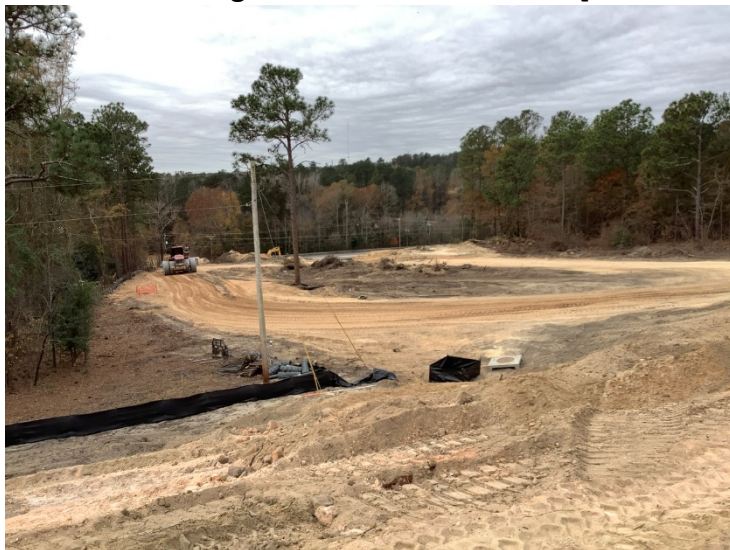
Site – View looking West toward Detention Pond 1 [12.07.2021]
