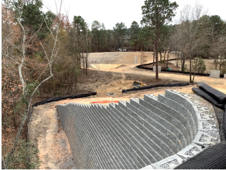
Site – View looking South – Detention Pond 3 [12.07.2021]
