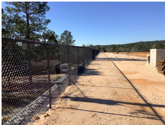
Site – South retaining wall view west [01.04.2022]
