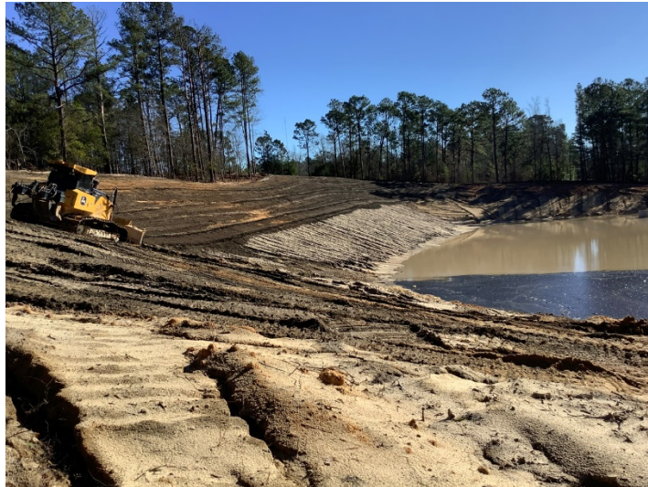
Site – View looking West - Detention Pond 1 [01.04.2022]
