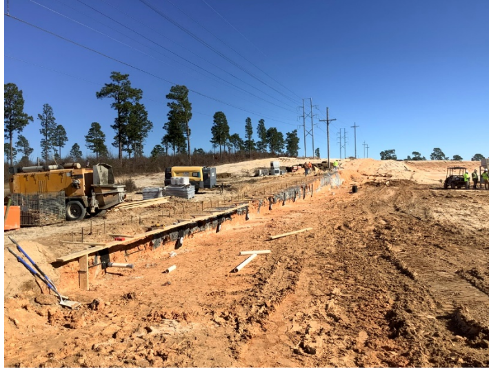
Site – North Retaining Wall – view looking east [01.04.2022]
