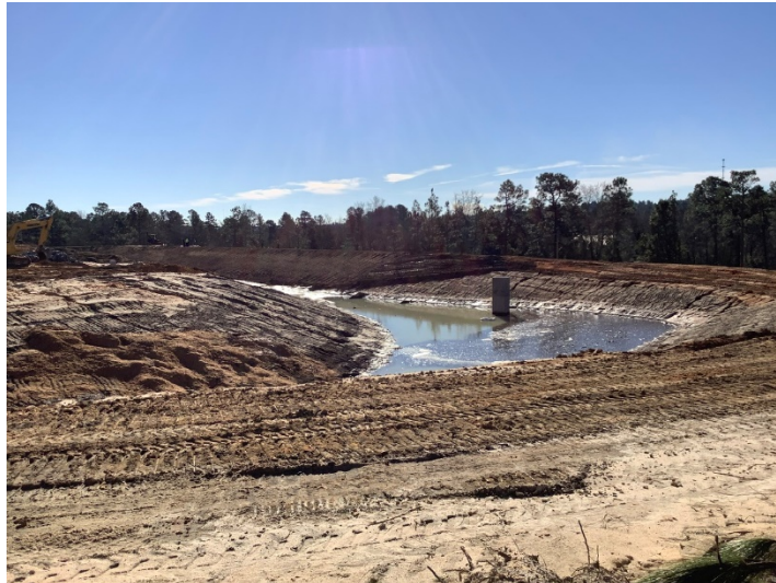
Site – View looking South – Detention Pond 2 [01.04.2022]
