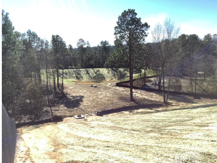
Site – View looking South – Detention Pond 3 [01.04.2022]
