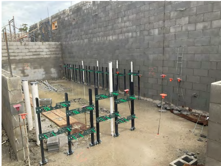
Area "D" Plumbing rough-in [05.24.2022]
