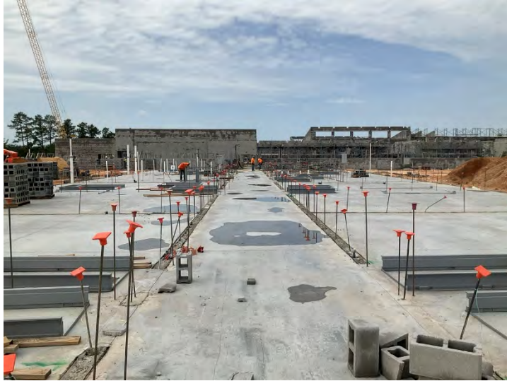
Area "C" slab-on-grade [05.24.2022]
