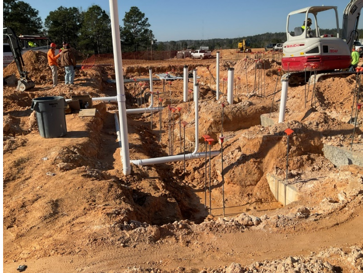
Plumbing & Electrical Rough-in Area "E" [02.01.2022]
