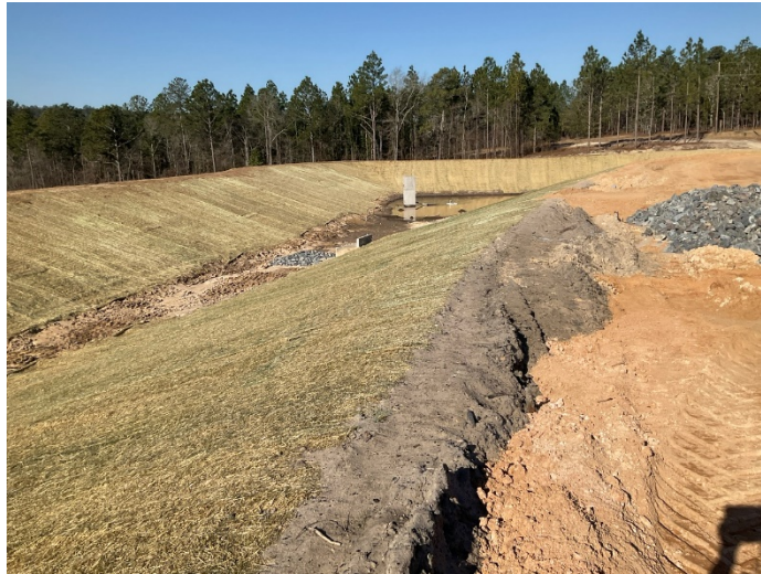
Site – View looking North – Detention Pond 2 [02.01.2022]
