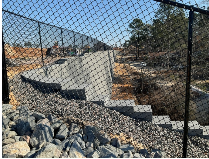
Site – South retaining wall view east [02.01.2022]
