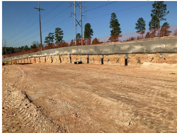
Site – north retaining wall [02.01.2022]
