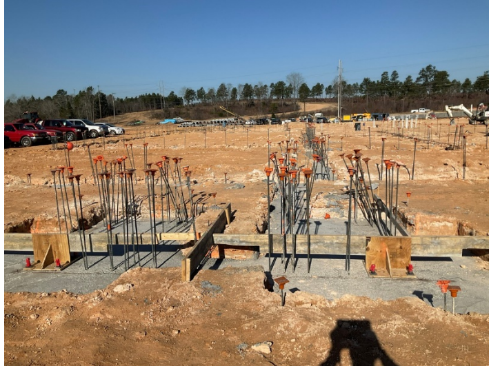
Foundations Area "E" [02.01.2022]
