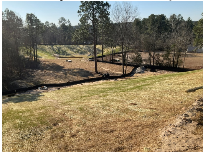
Site – View looking South – Detention Pond 3 [02.01.2022]
