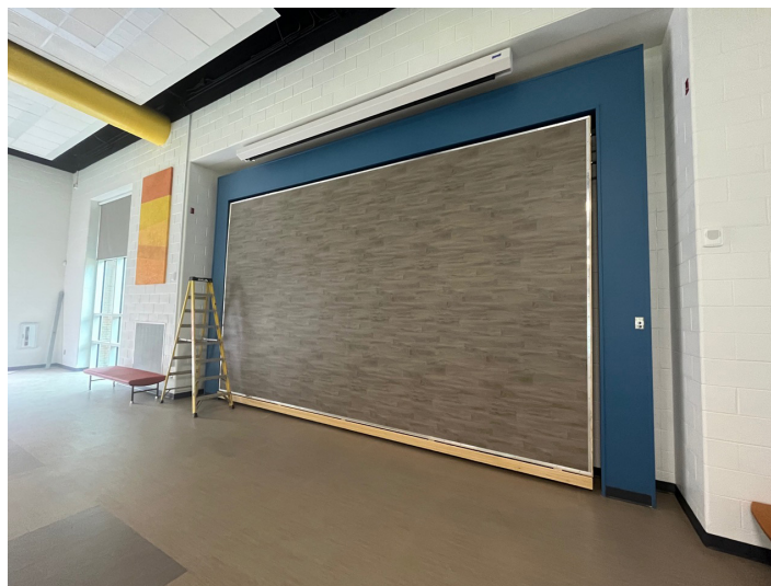
FINISH FLOORING INSTALLED ON RETRACTABLE STAGE.
