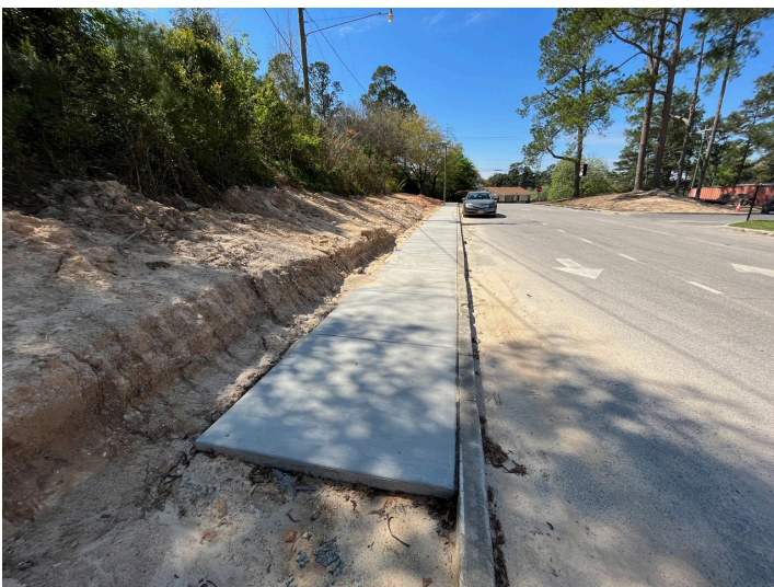
NEW SIDEWALK FROM WOODLAWN AVE. POURED.
