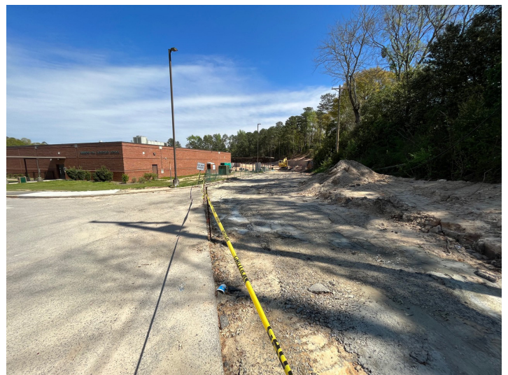
EXISTING ROADWAY BEING WIDENED.
