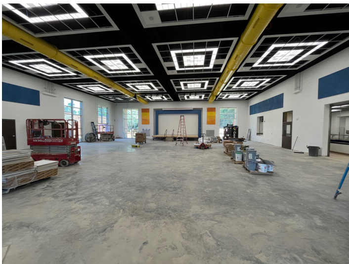
PHASE 2 INTERIOR CONSTRUCTION PROGRESS
