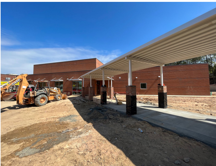
ALUMINUM CANOPY CONNECTOR INSTALLED.
