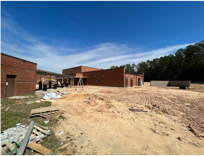
PHASE 2 EXTERIOR CONSTRUCTION PROGRESS
