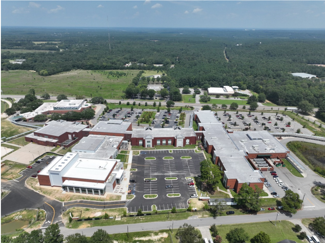
Aerial view North [08.16.2023 courtesy HGR]
