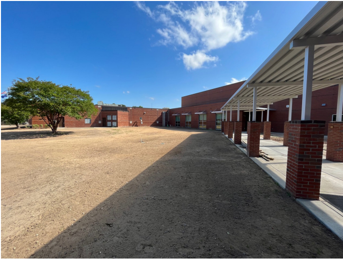
PHASE 2 SITE WORK PROGRESS
