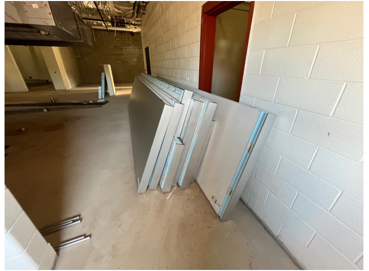
COOLER/FREEZER PANELS READY FOR INSTALLATION
