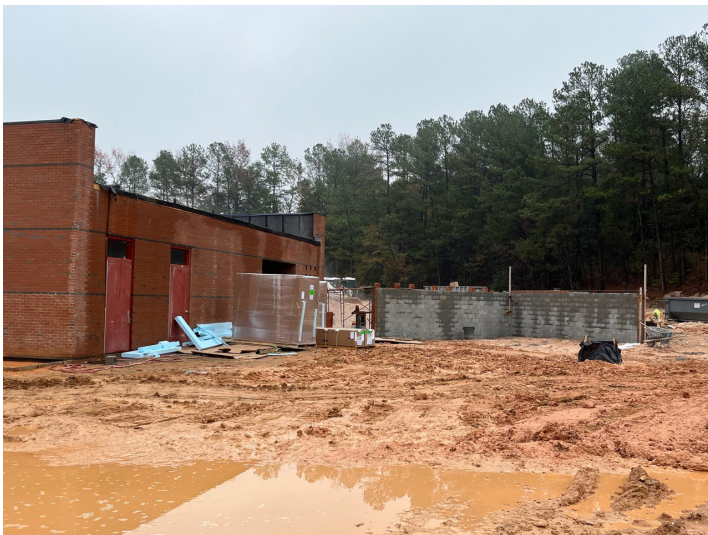
NEW DUMPSTER SCREEN WALL
