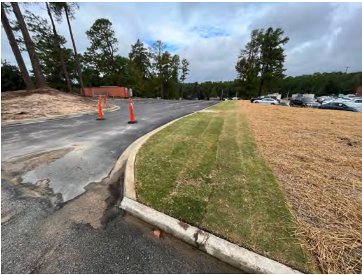
SODDING, GRASSING & IRRIGATION ON EACH SIDE OF VEHICULAR QUEING LANES COMPLETED.
