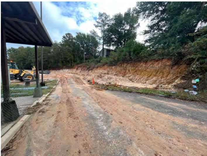
LOWERING OF ROADWAY & EXCAVATION OF HILLSIDE IS STILL IN PROGRESS
