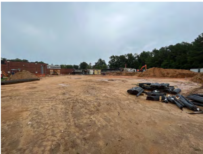
BUILDING PAD FOR PHASE 2 CONSTRUCTION GRADED & NEW FOOTINGS BEING DUG
