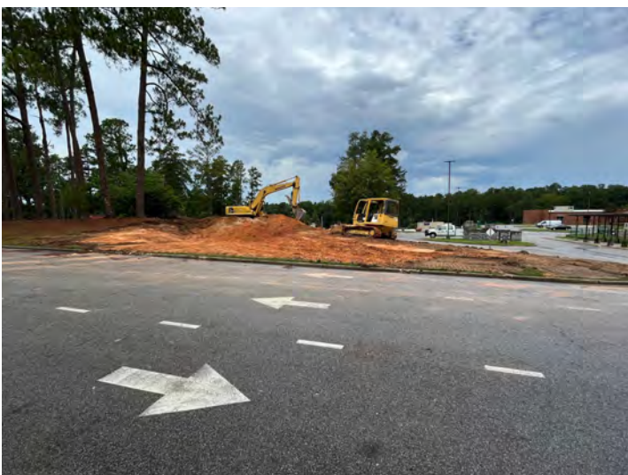
GRADING FOR NEW VEHICULAR QUEING LANES HAS STARTED
