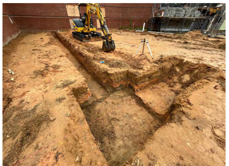
BUILDING PAD FOR PHASE 2 CONSTRUCTION GRADED & NEW FOOTINGS BEING DUG
