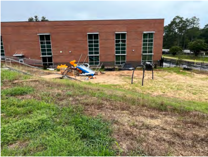
PLAYGROUND INSTALLATION IN PROGRESS
