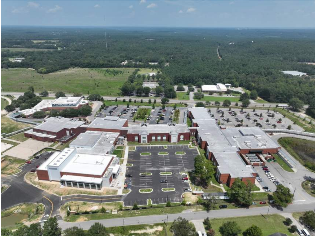
Aerial view North [08.16.2023 courtesy HGR]
