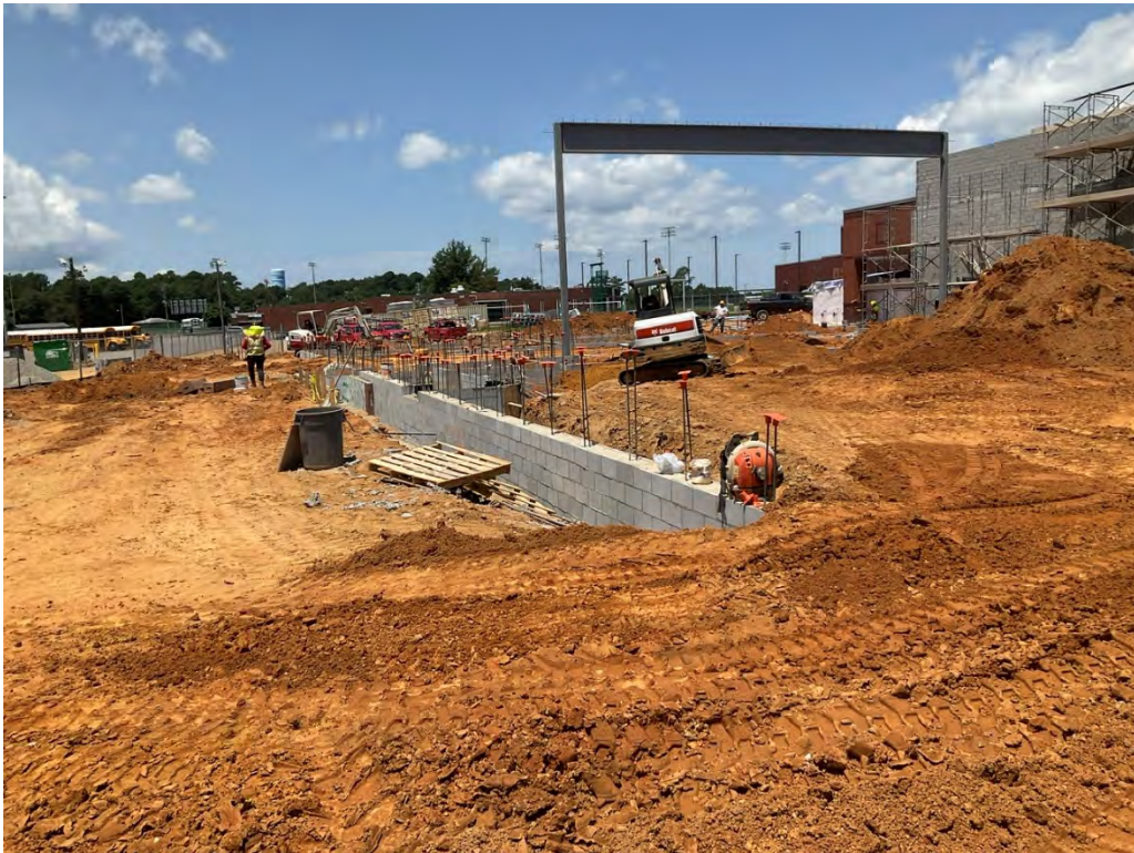
Below-slab CMU, Stage steel [07.19.2022]
