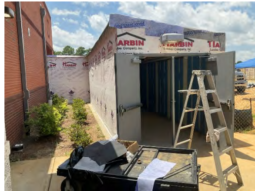
Temp. Egress Tunnel Discharge [07.19.2022]
