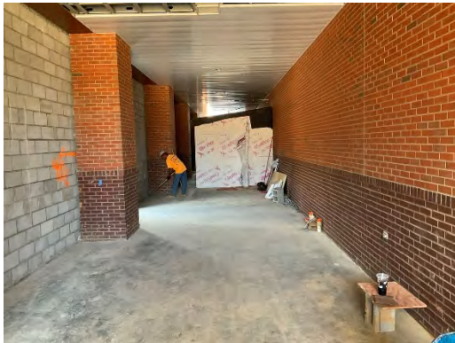
Temp. Egress Tunnel at Existing [07.19.2022]
