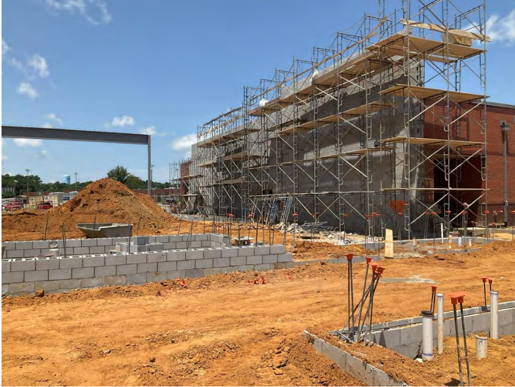
Site – view West [07.19.2022]
