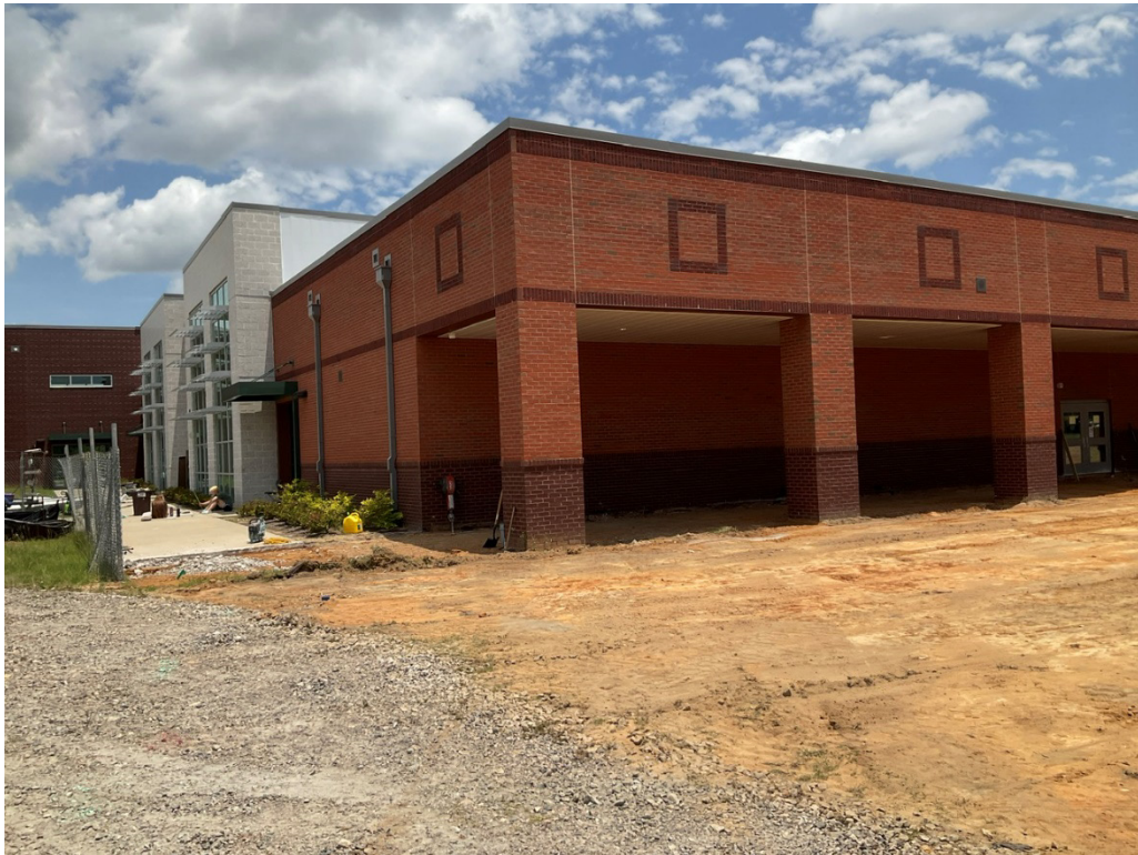
Existing Building – view Northeast [06.07.2022]
