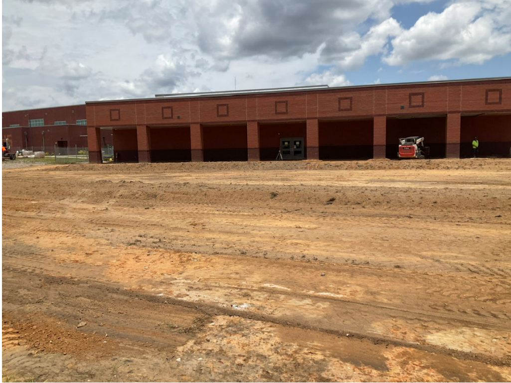
Site – view South [06.07.2022]
