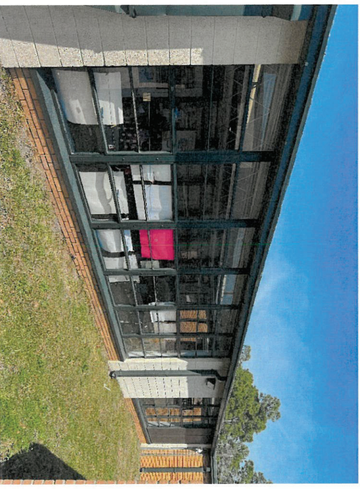
EXISTING STEEL WINDOWS W/ SINGLE PANE GLASS
