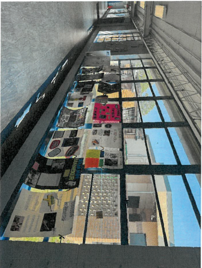
EXISTING STEEL WINDOWS W/ SINGLE PANE GLASS
