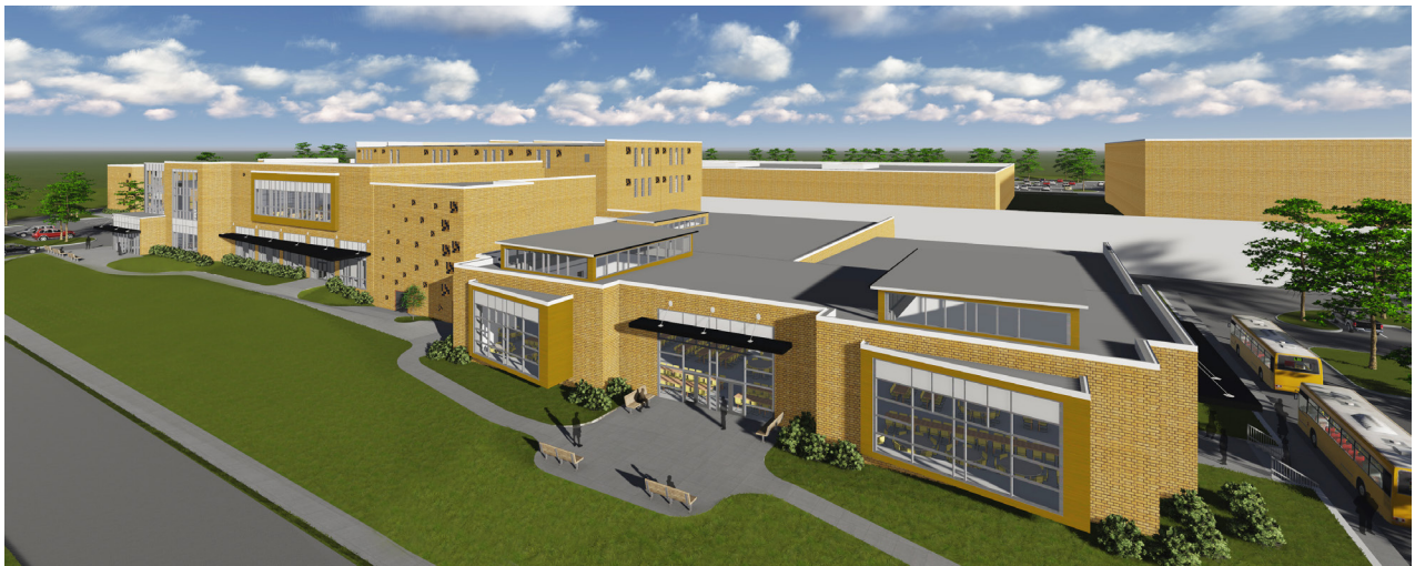
View Looking East
