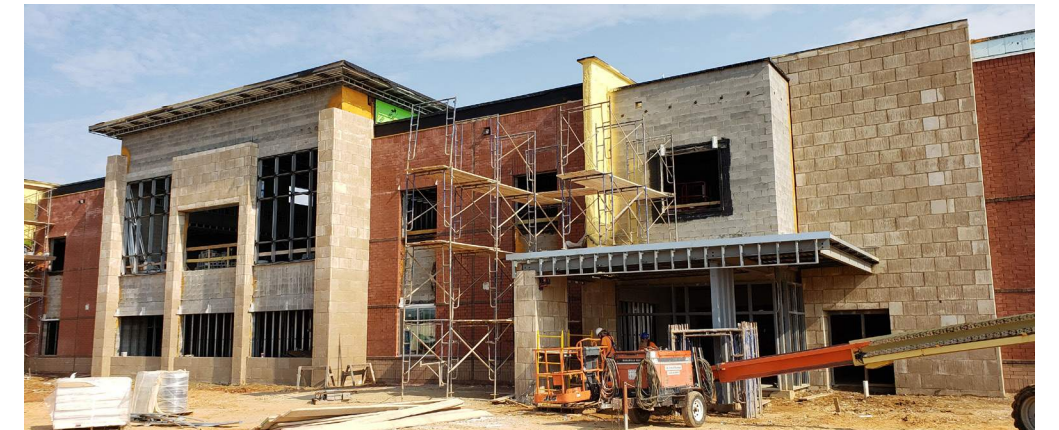
MAIN ELEMENTARY SCHOOL ENTRY UNDER CONSTRUCTION
