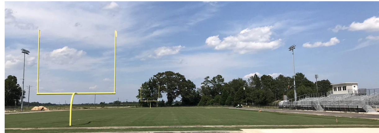
FOOTBALL/TRACK STADIUM UNDER CONSTRUCTION
