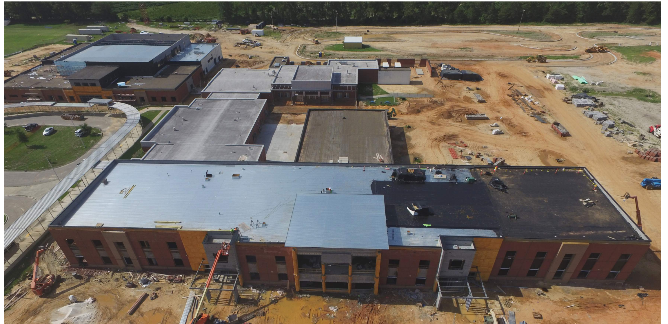
PHASE 2 CLASSROOM AND ACTIVITIES BUILDINGS UNDER CONSTRUCTION
