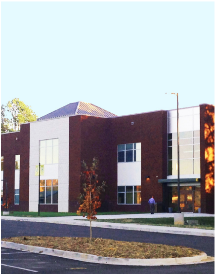
EXISTING SCIENCE BUILDING TO REMAIN
