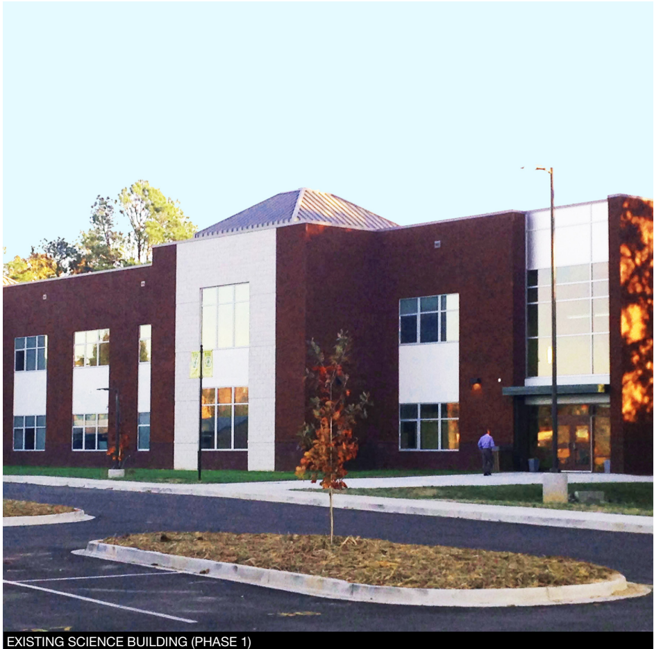
EXISTING SCIENCE BUILDING (PHASE 1)
