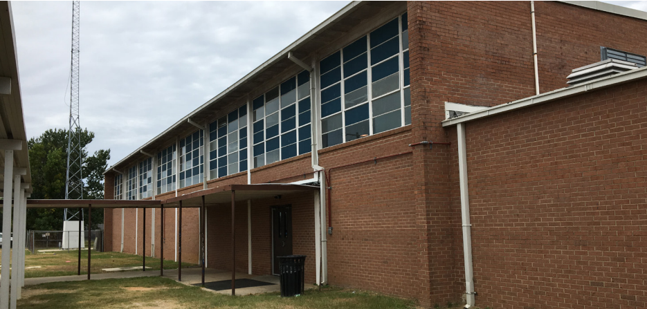
EXISTING GYMNASIUM BUILDING
