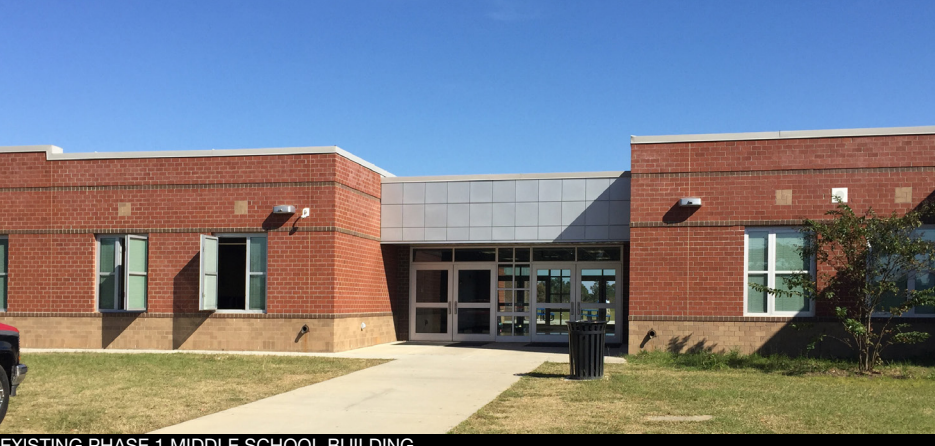
EXISTING PHASE 1 MIDDLE SCHOOL BUILDING
