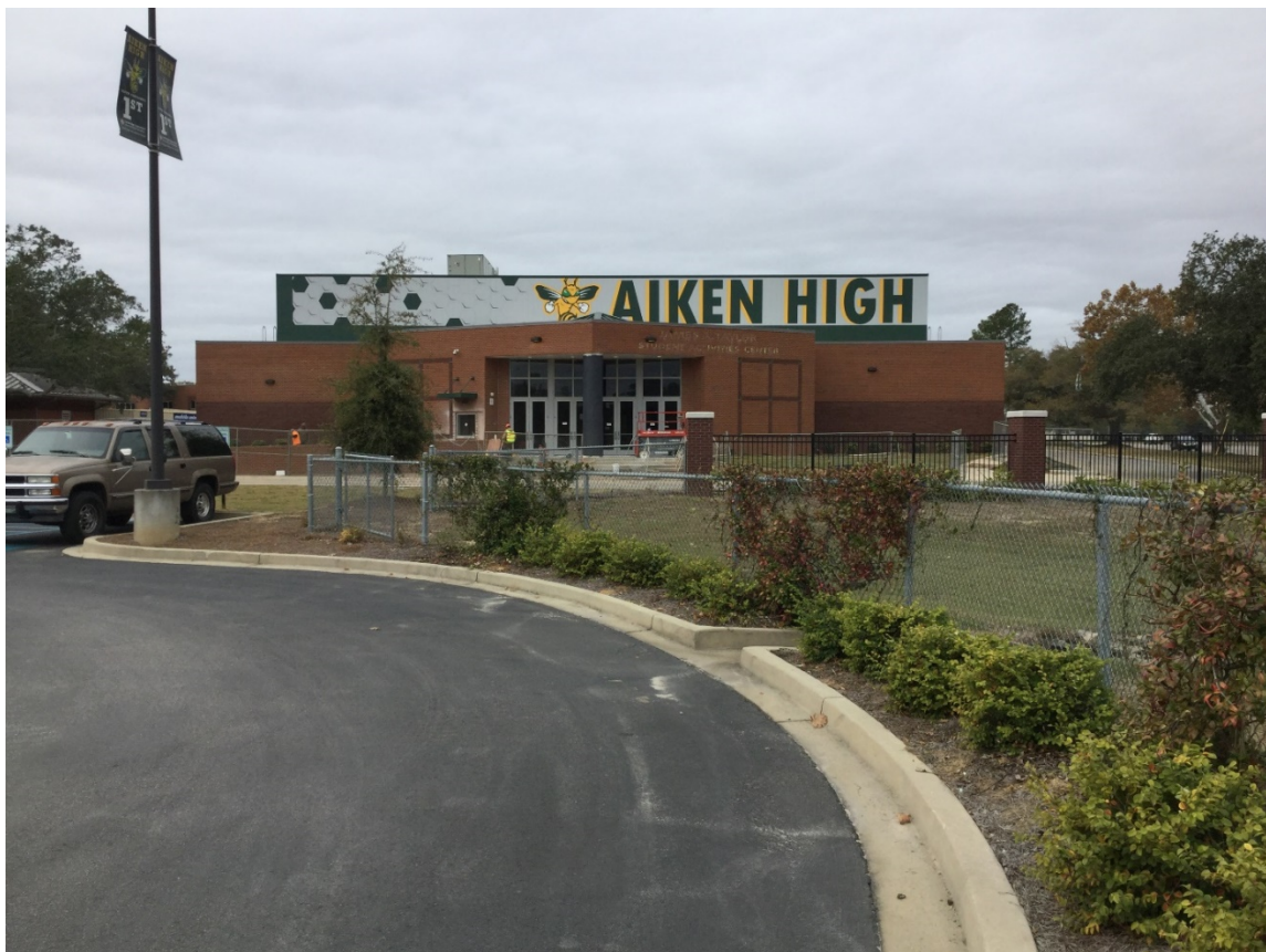
Exterior metal panel graphic installed.
