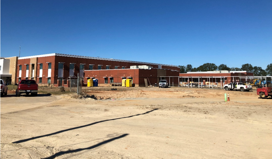
Area "A": Classroom Addition
