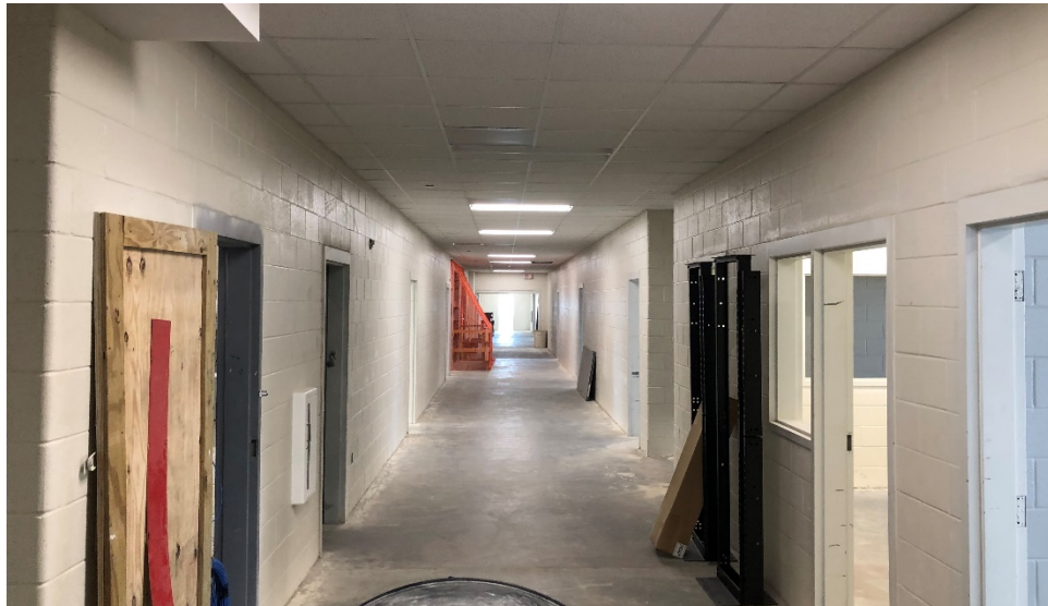
Area "B" – 2 nd Floor Corridor
