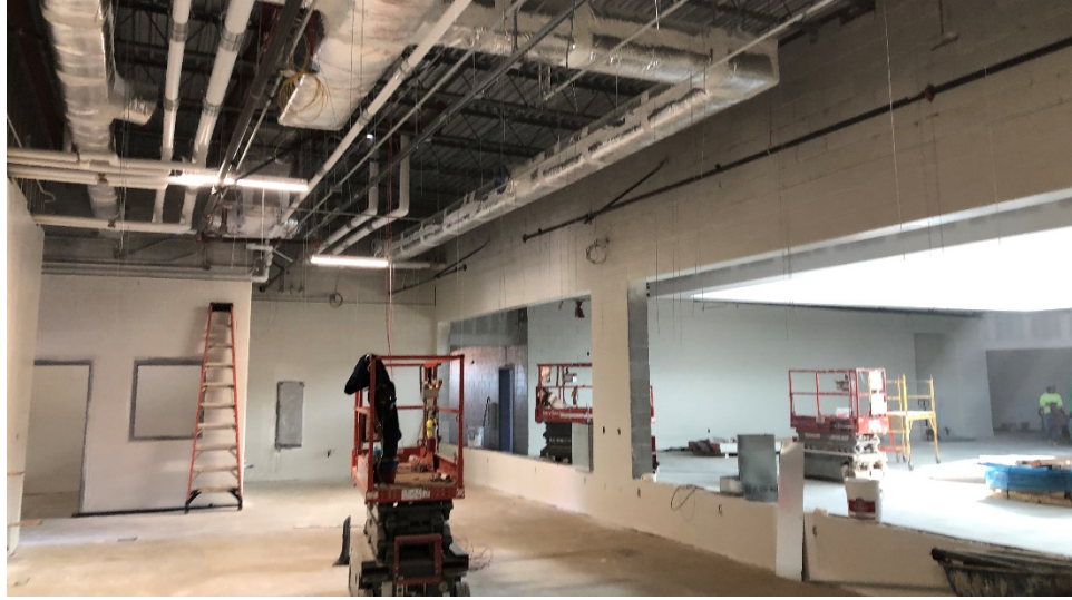
Area "C" – Kitchen and Serving Line
