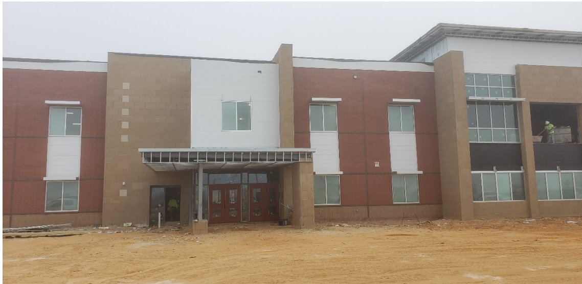
Area “A” – Front Elevation (Main Entry)
