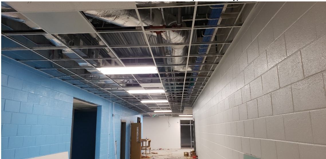
High School – First Floor Corridor A101B
