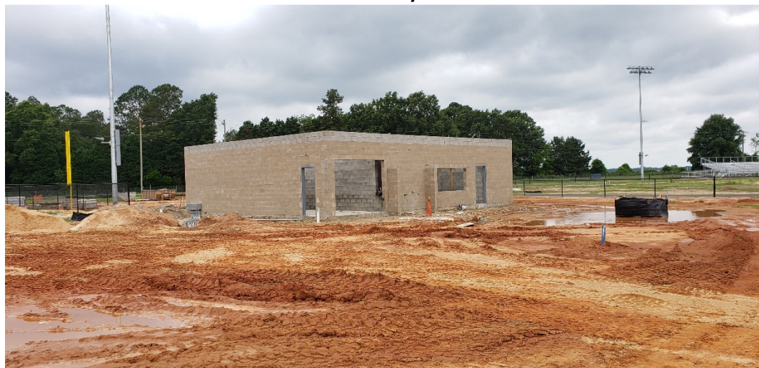
Athletic Fields – Concession Stand & Restrooms
