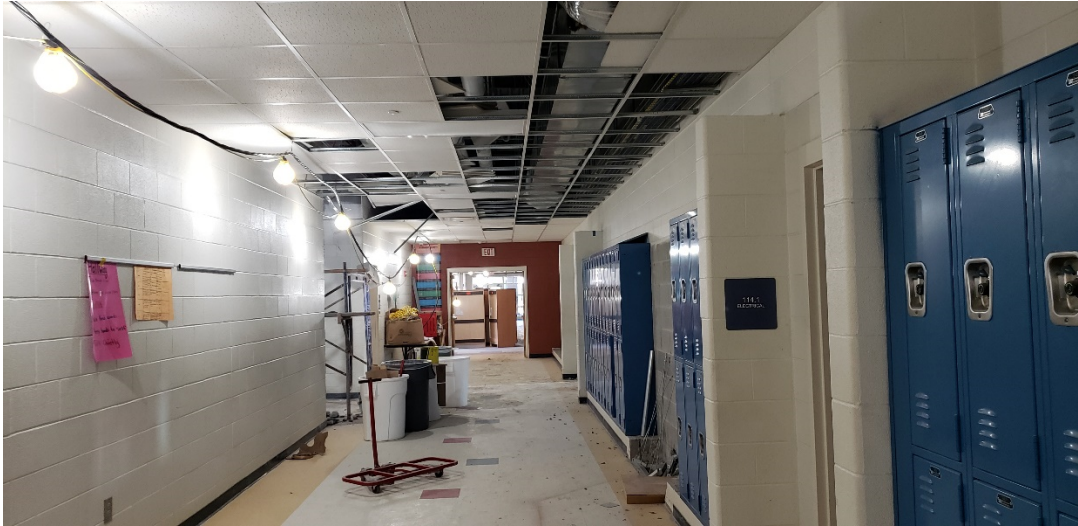
Area "C" – Existing Middle School Demolition
