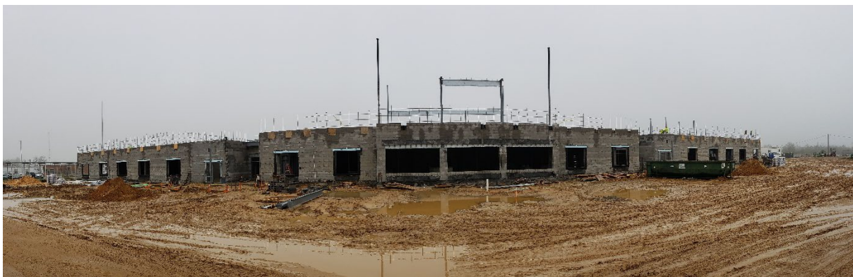
Area “A” – Front Elevation / Entry
