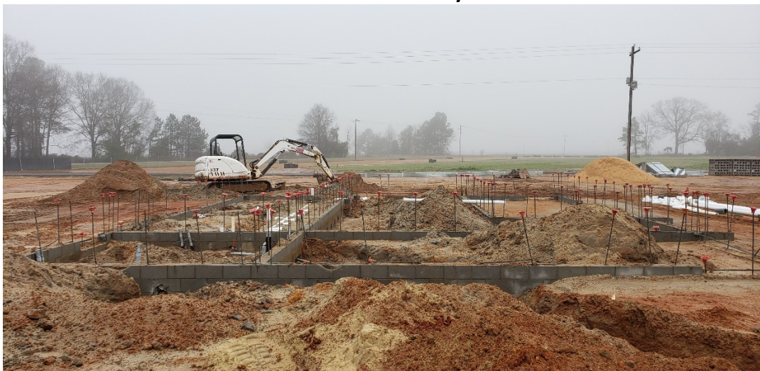
Concessions Building - Footings
