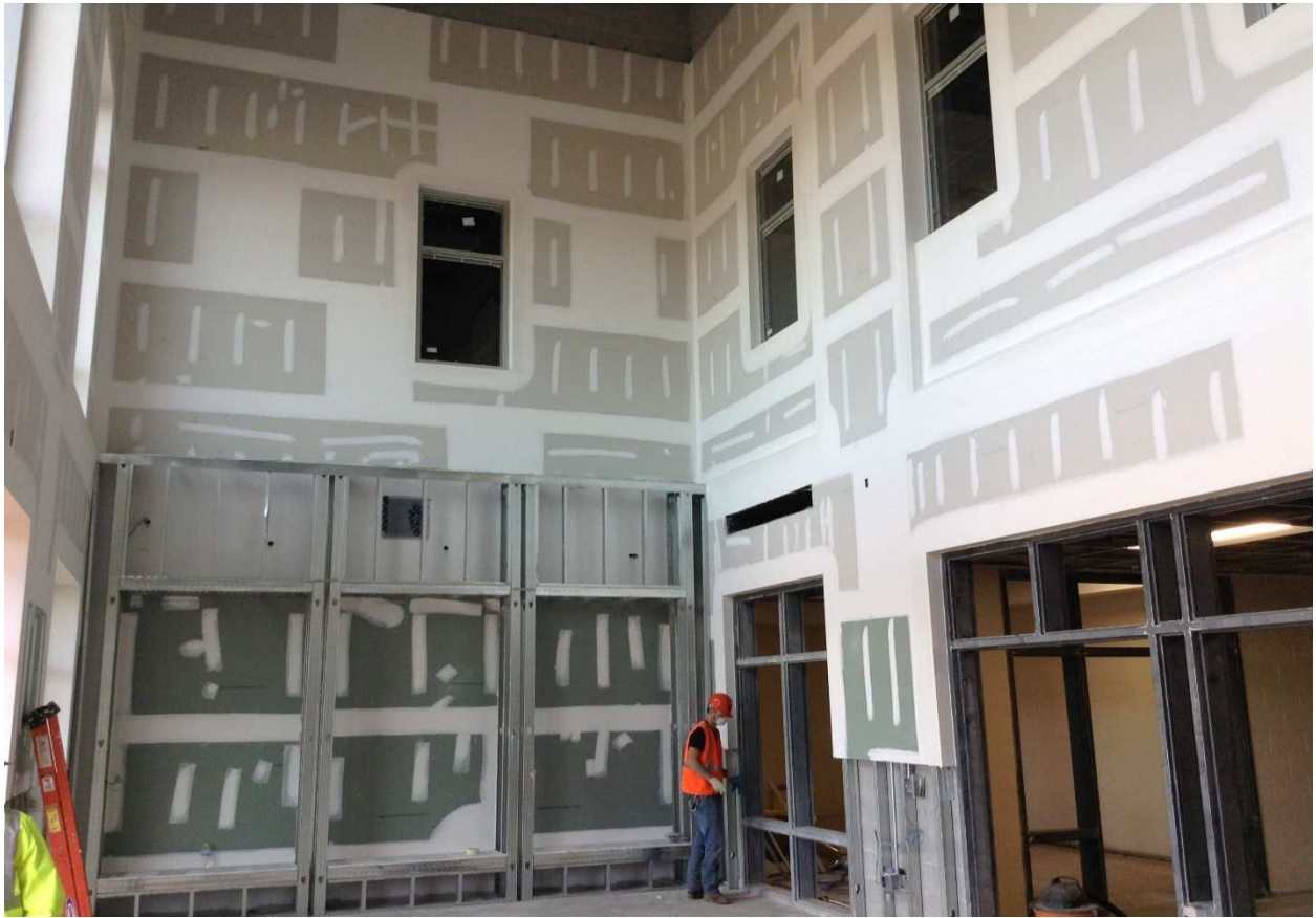
Finishing sheetrock main entrance vestibule
