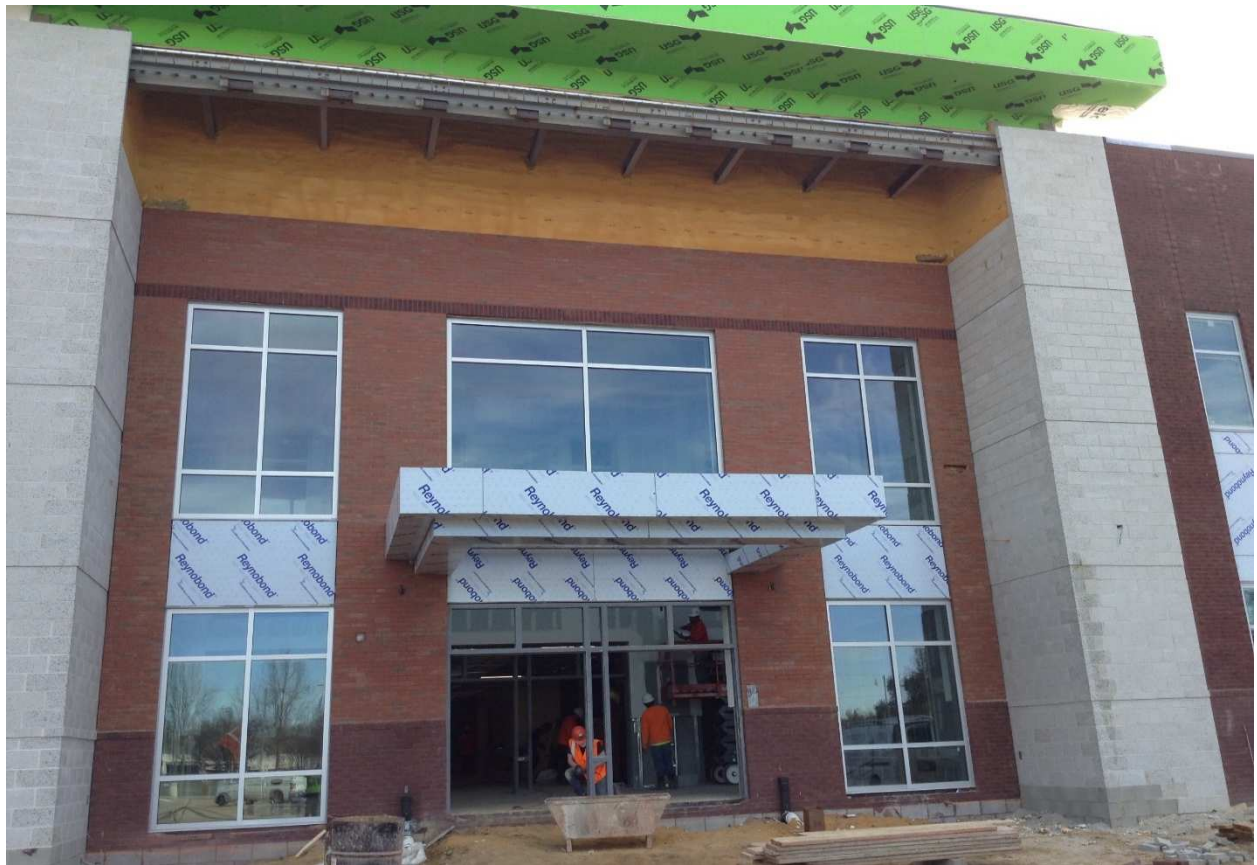
Main entrance windows and ground face block complete
