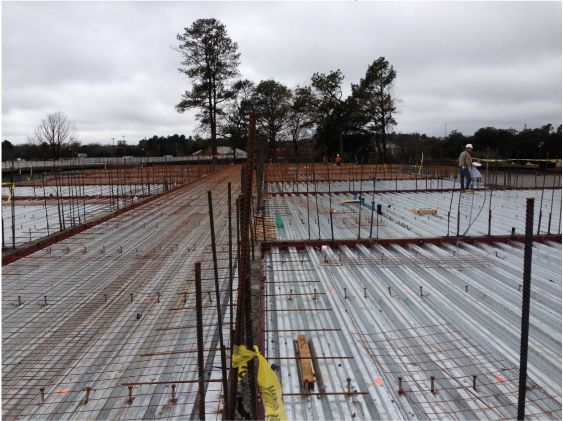
Science Classroom Wing
