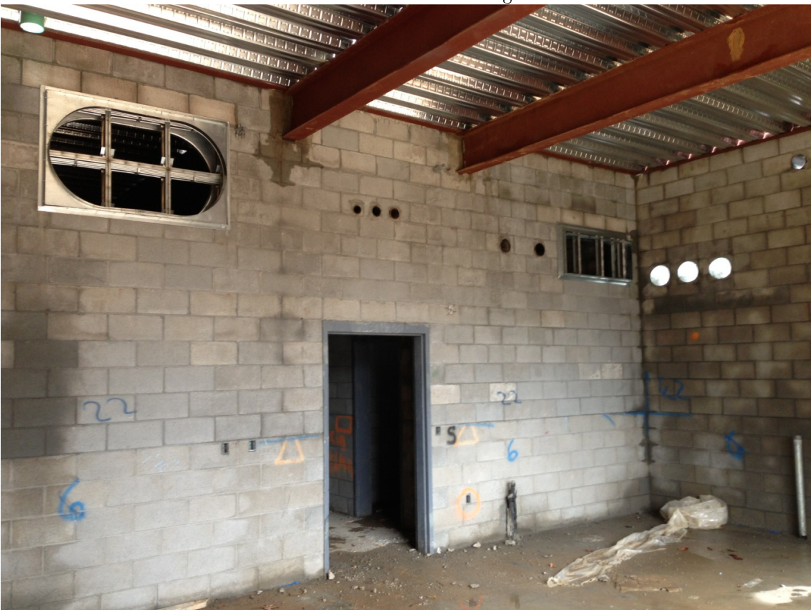
Science Classroom Wing
