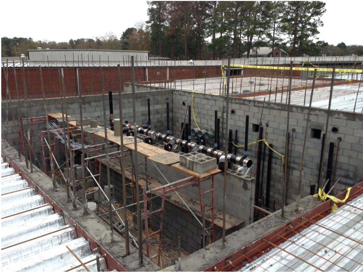
Science Classroom Wing
