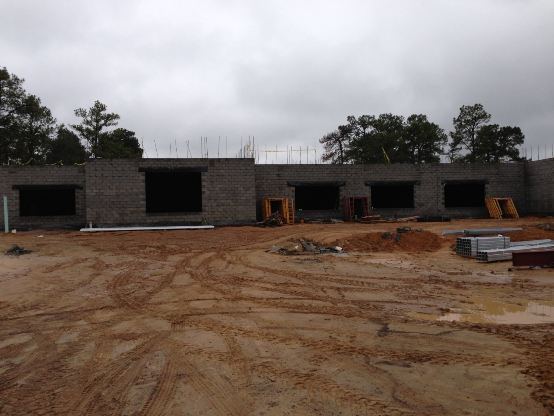
Science Classroom Wing
