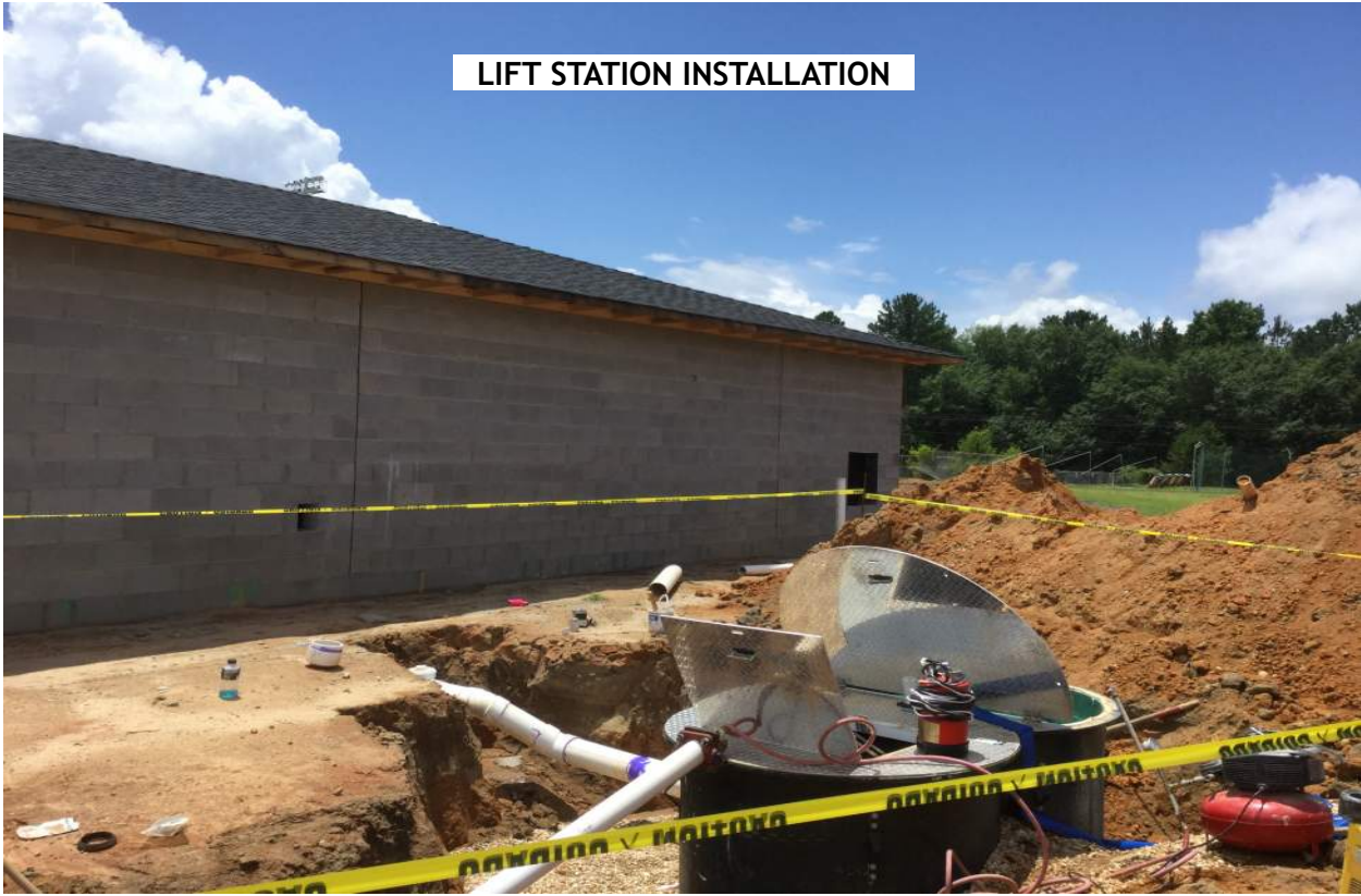
LIFT STATION INSTALLATION
