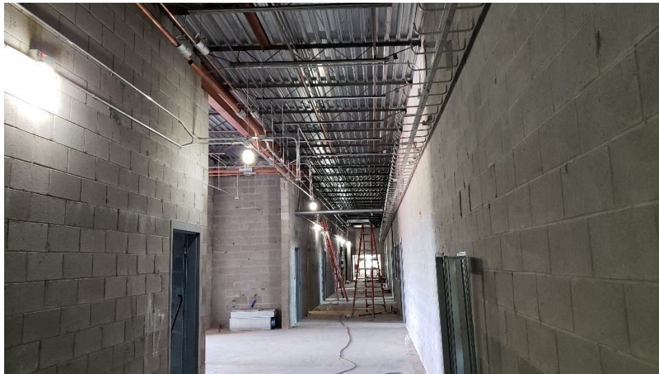
Area "B" – Second Floor Corridor
