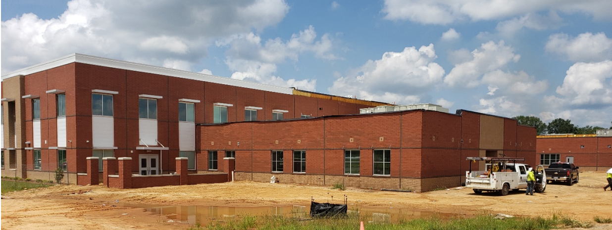
Area "A": Classroom Addition
