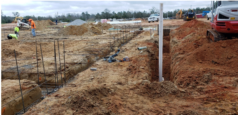
Footings and plumbing underground rough-in
