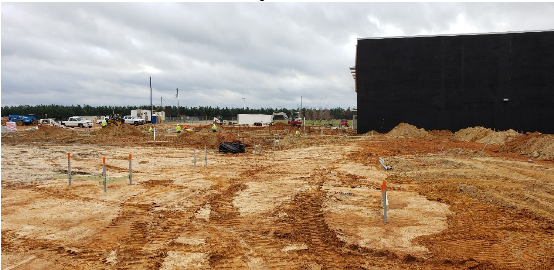
Building layout and footing excavations
