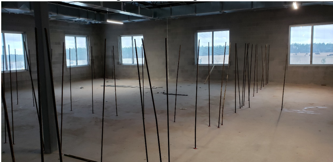
Wall layout & rebar in Phase 2 Shell space
