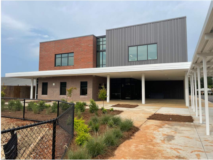
Exterior progress photo.
