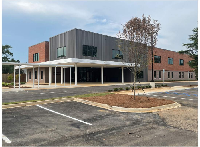
Exterior progress photo.
