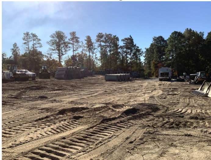
Site – View looking South
