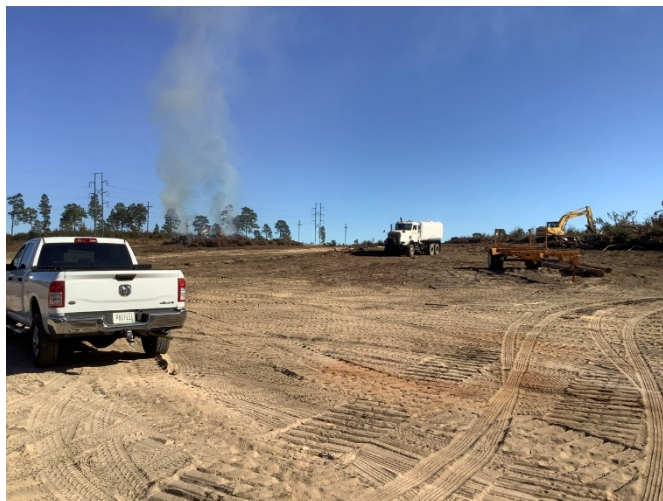
Site – View looking North
