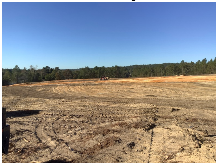
Site – View looking West
