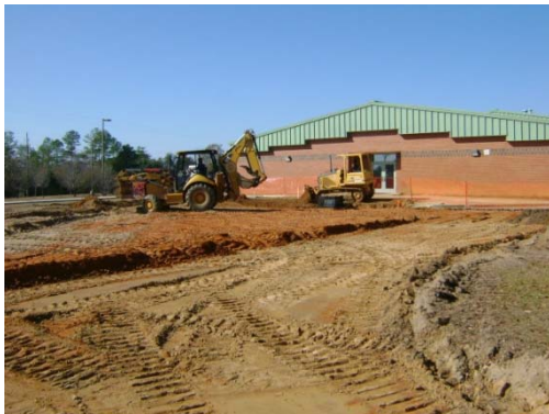
Site preparation, classroom wing beyond
