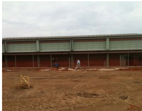
Site preparation, gymnasium beyond
