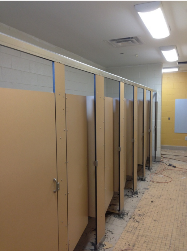
Toilet Partitions and Sinks Installed
