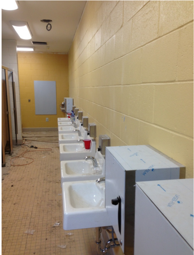
Toilet Partitions and Sinks Installed
