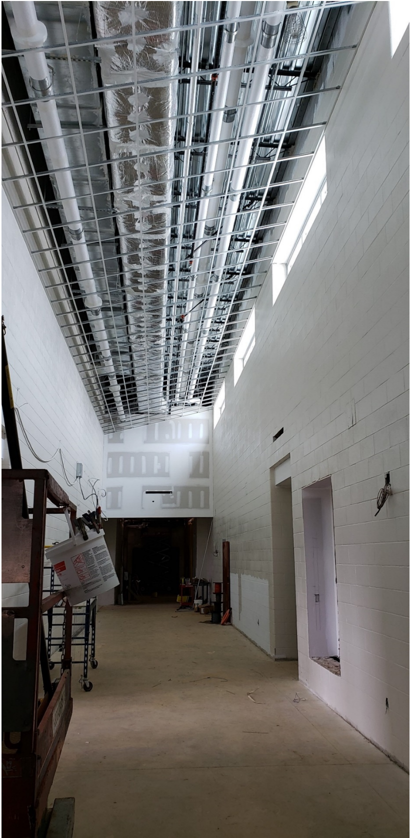
Ceiling grid in corridor of ROTC/Band Building
