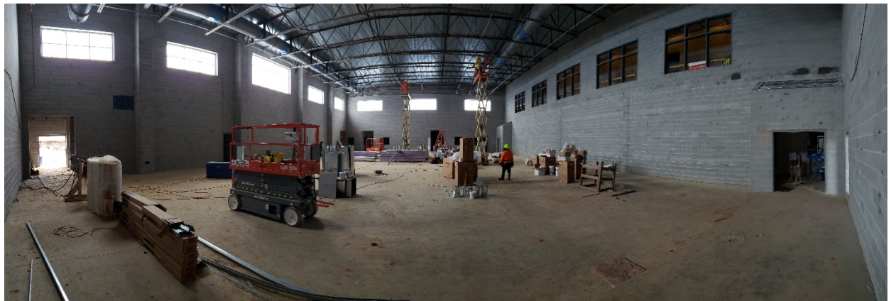
Overhead rough-ins at gym
