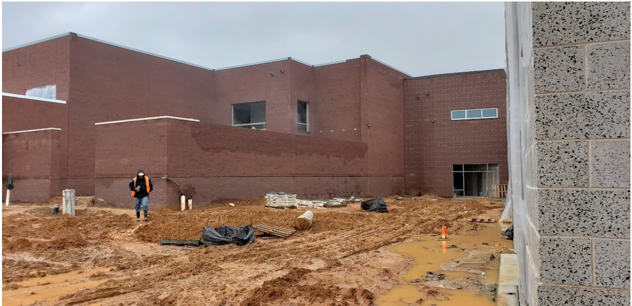
Majority of masonry veneer complete
