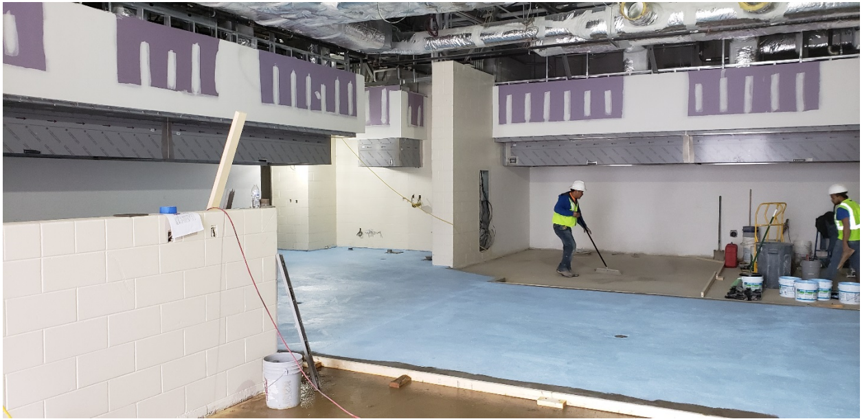
Kitchen hoods and topping slab in Culinary Arts
