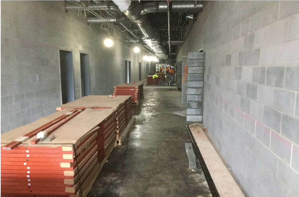
Corridor at front classroom with above ceiling rough-in
