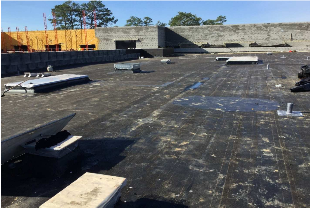
Roof dry-in above cafeteria
