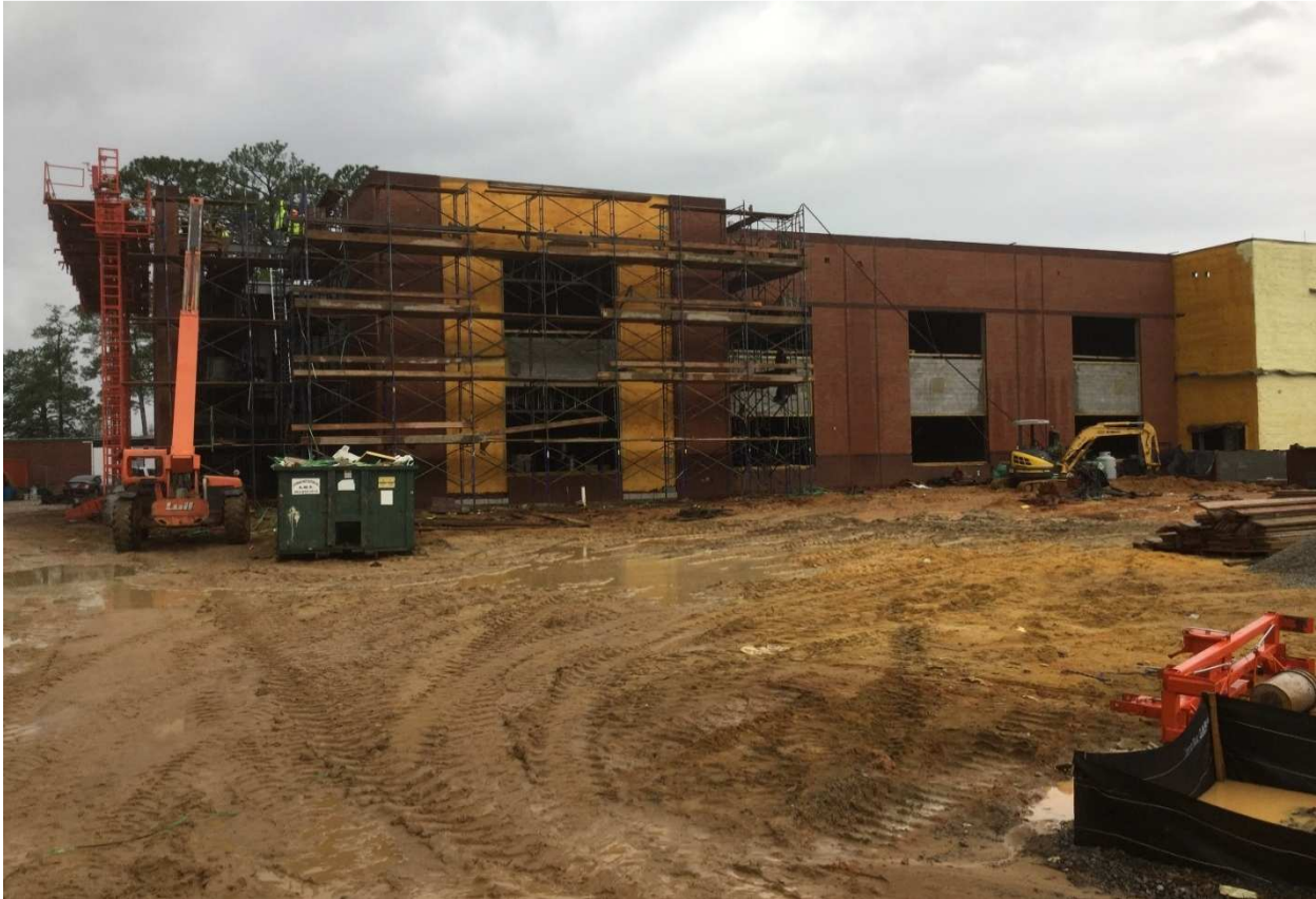
Brick veneer at front classroom wing
