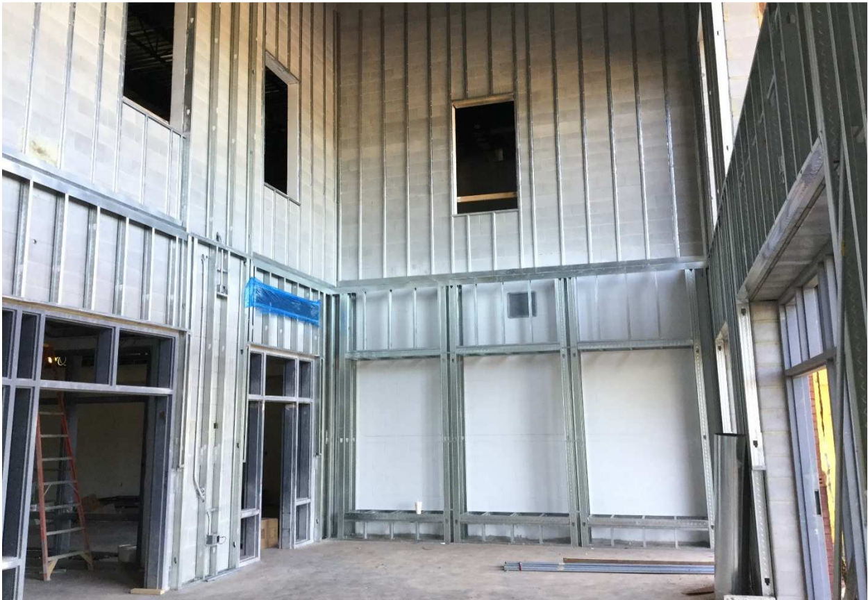
Wall framing at entrance vestibule to admin building
