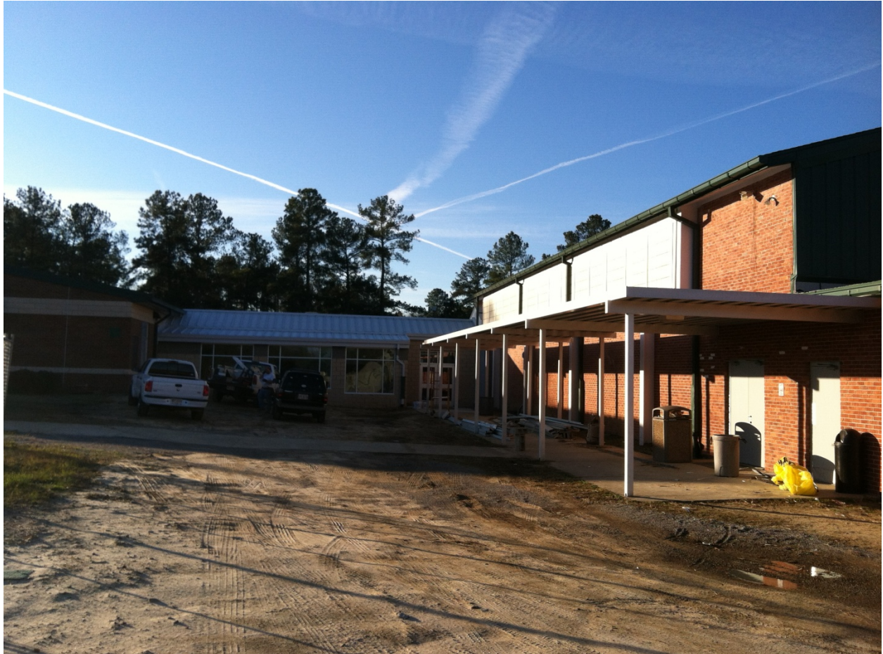
1 – Addition viewed from the north. Final grading and grassing, extension of walk cover are not complete.
