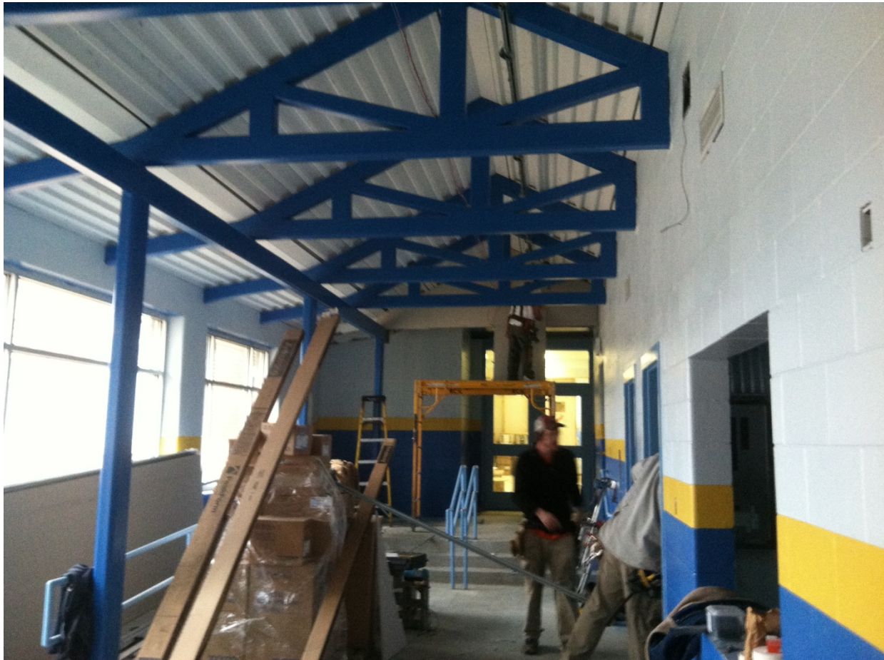
2- Addition interior from the gymnasium. Color scheme was changed to match the interior colors that were used when the existing school was re-painted over the Summer of 2012.
