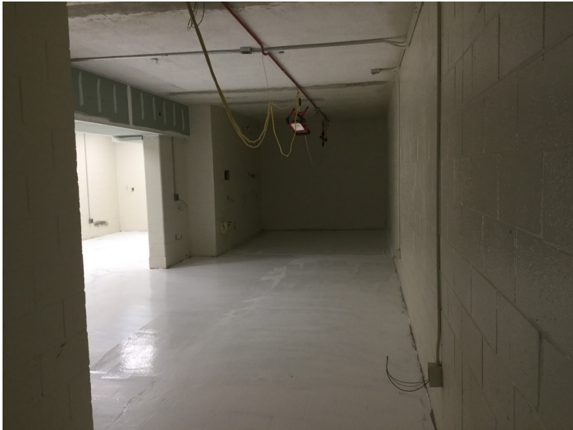
New epoxy floors in progress at training room.
