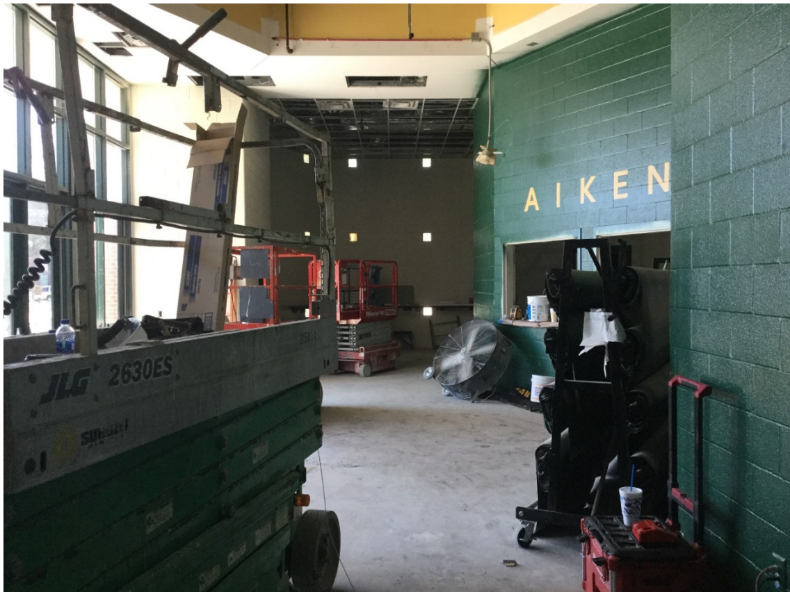
Above ceiling rough ins and paint at entrance lobby.
