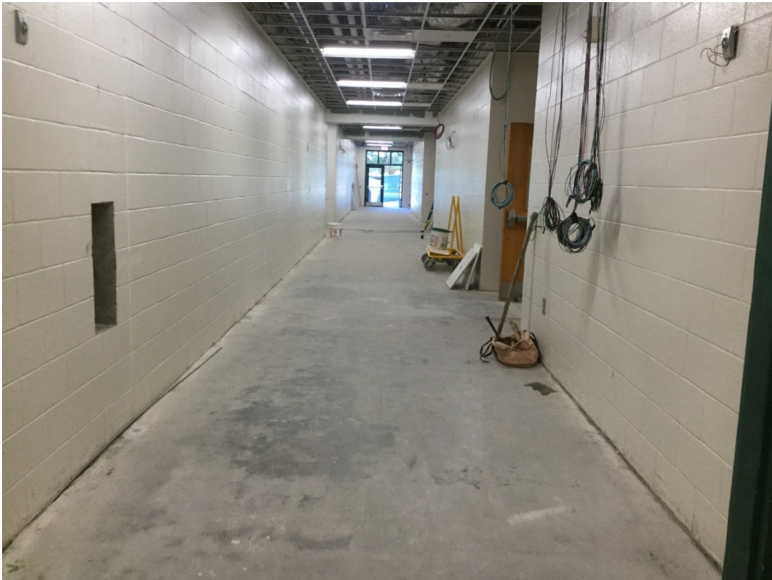
New grid and permanent lighting at weight room corridor.
