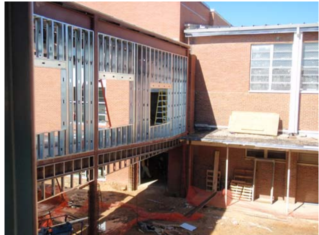
Framing of Connecting Corridor
