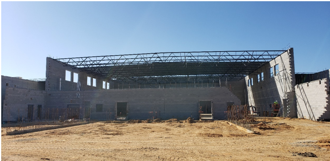
Area "D" – Main Gym (view looking south)
