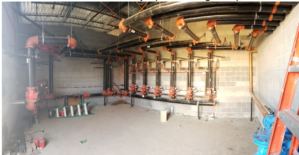
Area "C" – Main Fire Protection Room
