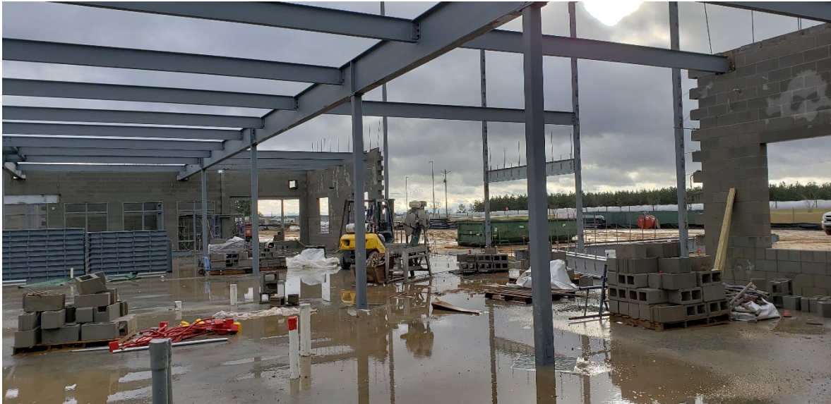
Area "A" – Steel Erection at Administration Area
