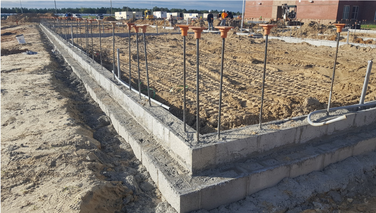
Area "B" Footings, Below-grade CMU
