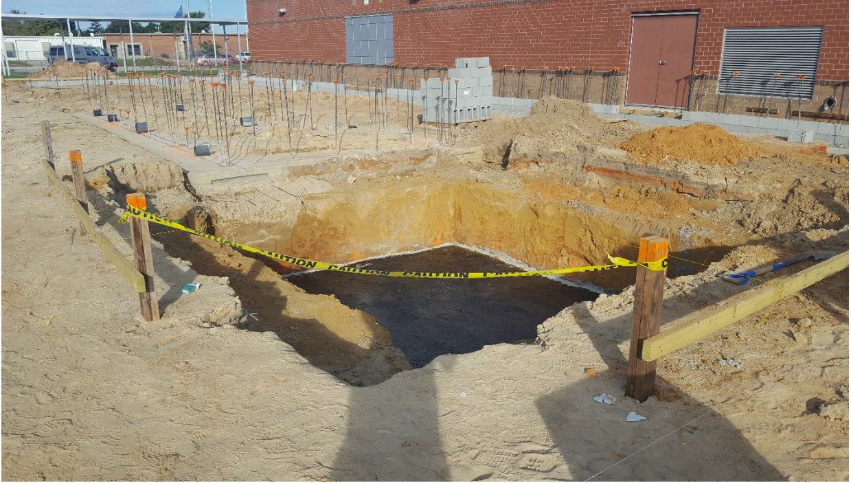
Area "A" footings, elevator pit
