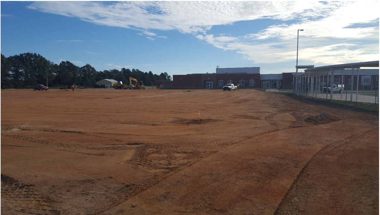
Area "D" building pad
