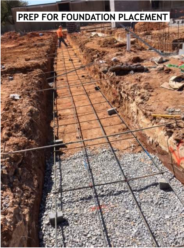
PREP FOR CONCRETE PLACEMENT
