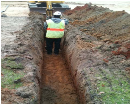
Special inspector in footing excavation
