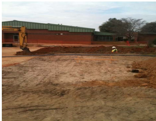
Excavating footings, South wall.
