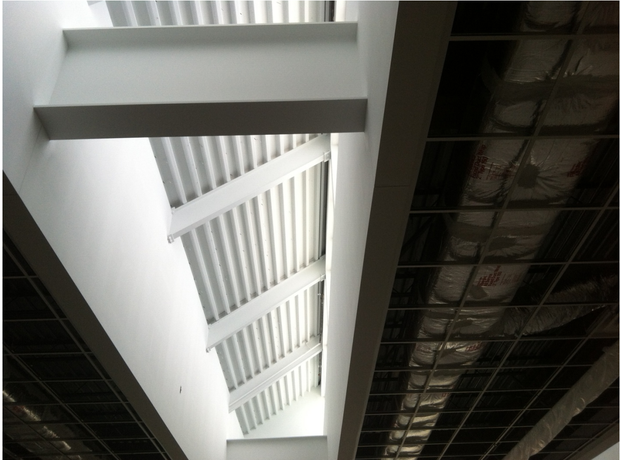
2 – Dining room interior clerestory windows in roof monitor.
