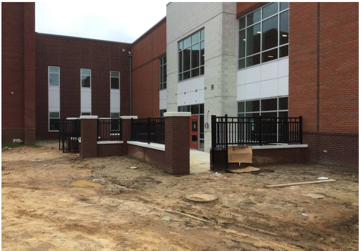
Brick wall and fence complete at media center courtyard
