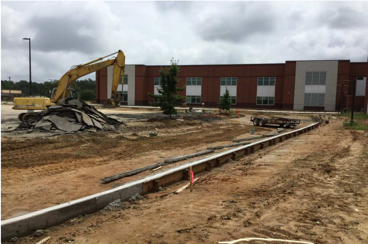
Sitework demo and new curb forms at front parking lot
