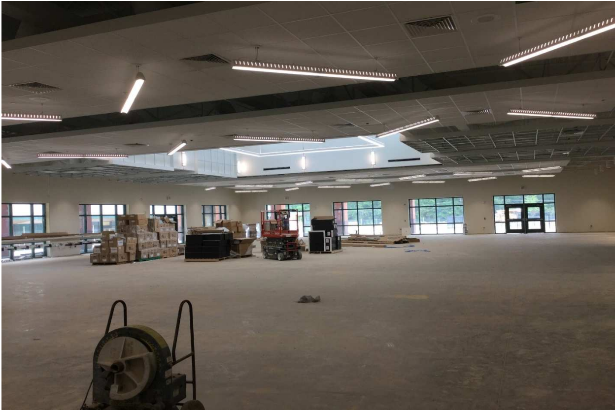
Permanent lighting at cafeteria dining
