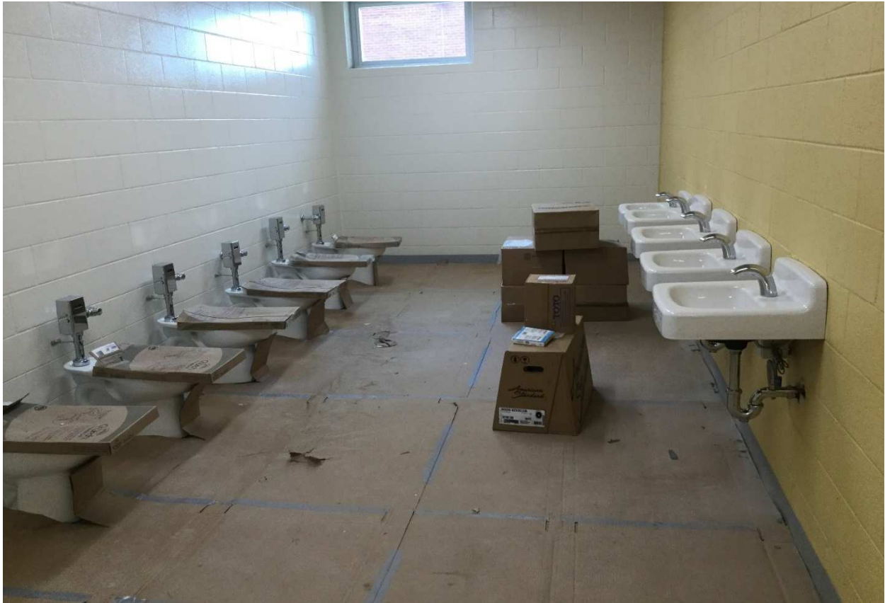
Toilet fixtures in bathrooms in rear Classroom wing A
