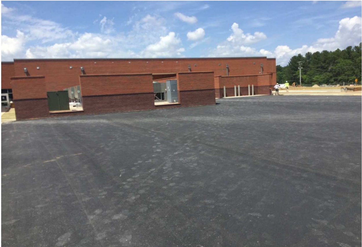
Asphalt pavement at loading dock area and bus loop road
