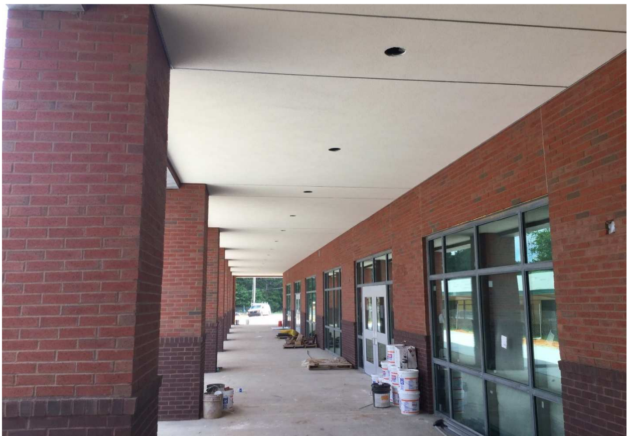
Ceiling and sidewalk finished along breezeway
