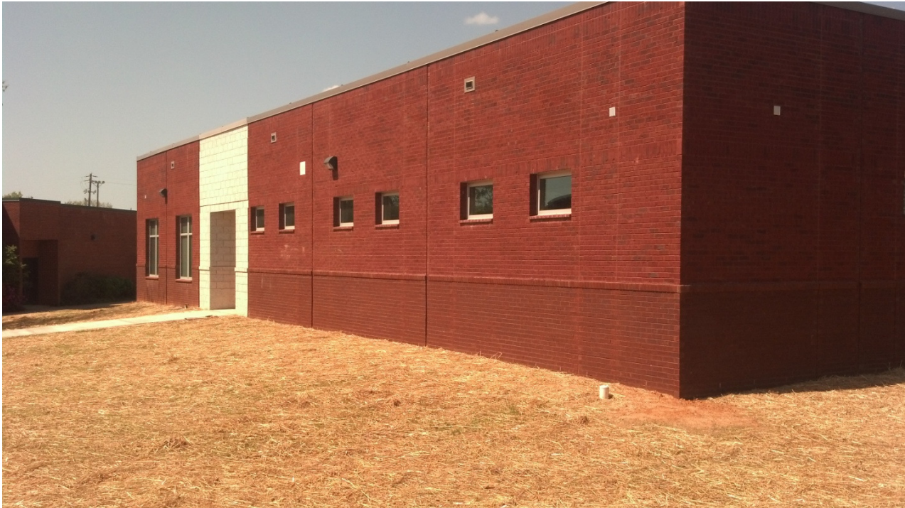
Field House Exterior
