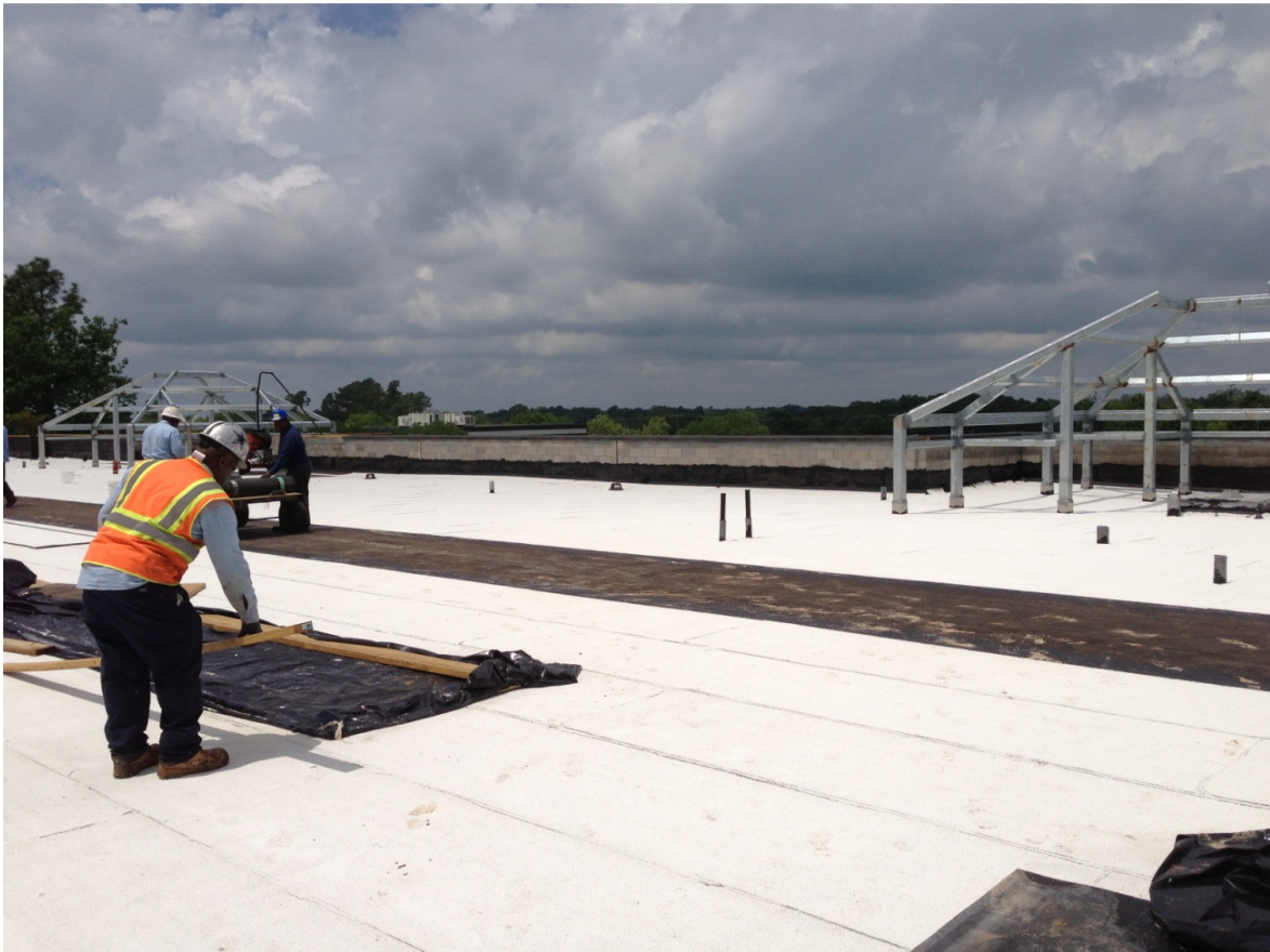
Science Building Roof
