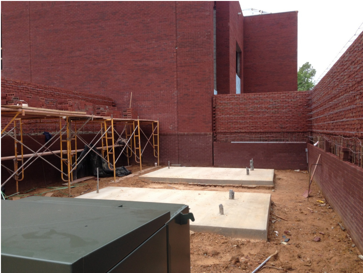
Screenwall at Science Building's Chiller
