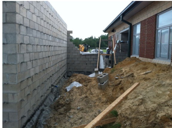
4- Connecting corridor to the existing classroom building on the right.
