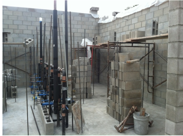
2– Boys rest room plumbing rough-in.
