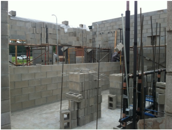
1 – Girls rest room plumbing rough-in. Concessions room and corridor beyond.
