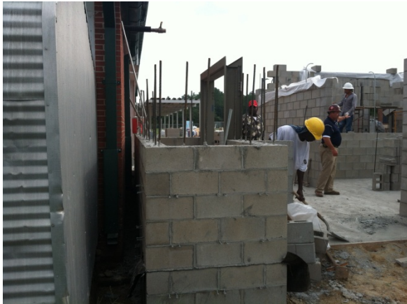
3- Fire wall construction next to the existing gym. Metal storage building is existing.
