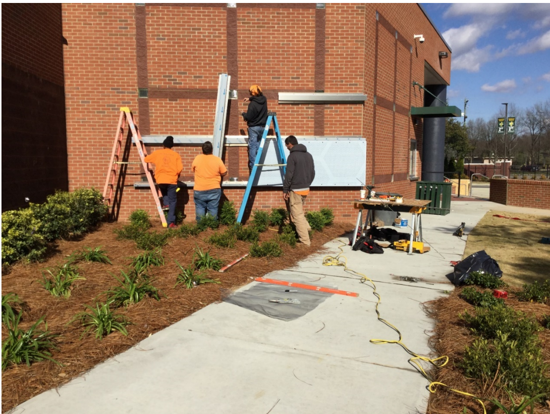
Metal wall panels in progress.
