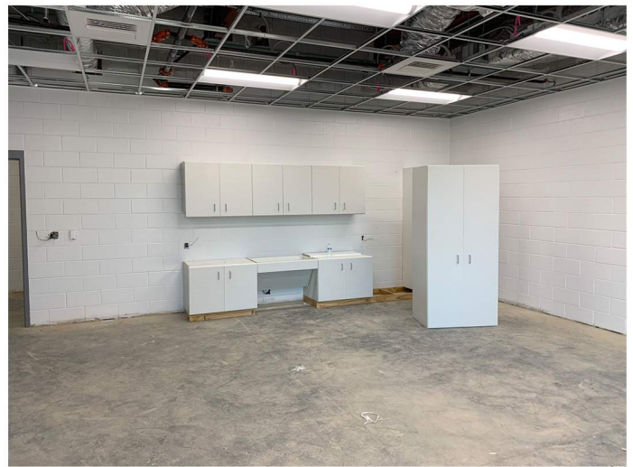
Millwork installation is in progress.
