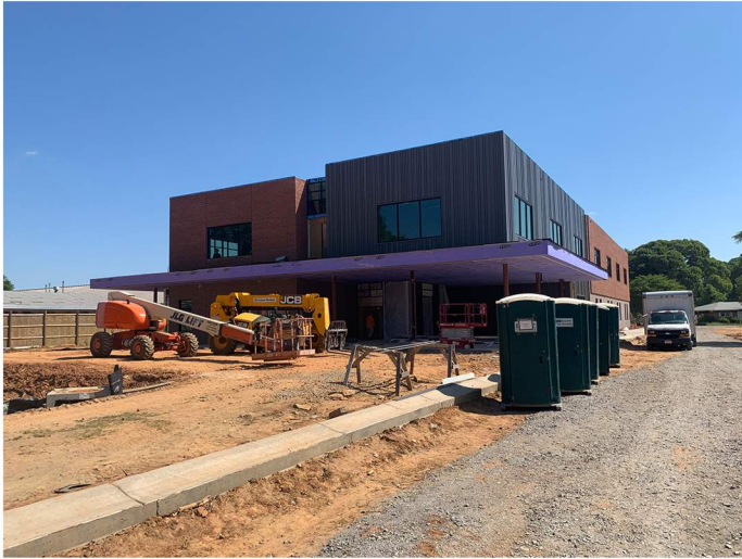
Exterior progress photo.
