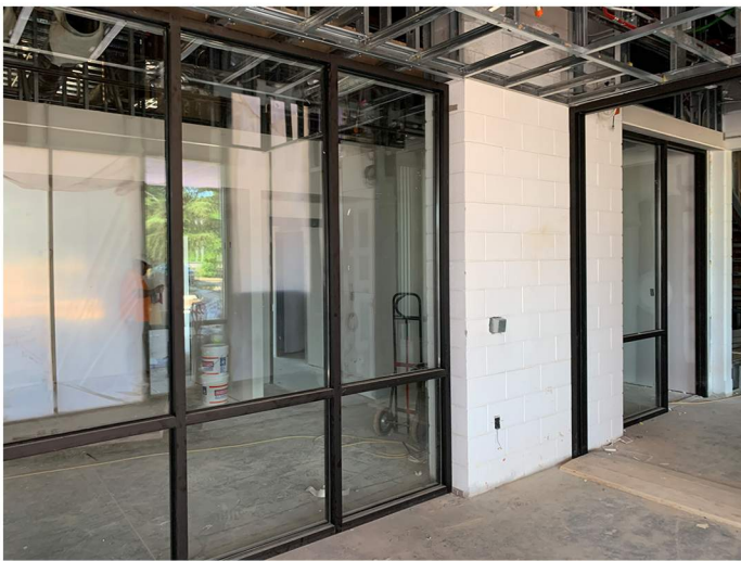
Storefront is largely complete.
