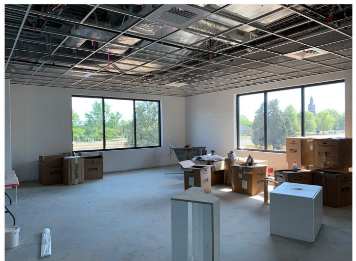
Typical second level classroom space.
